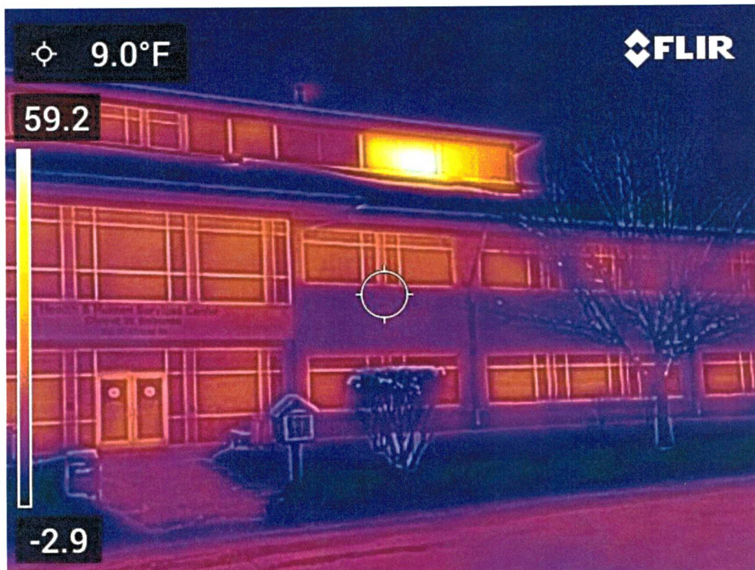
Figure 14. Thermal image of exterior enclosure of HHS facility (North Side- Chapel Street Entrance). Note the heat from the penthouse from the VRV Exhaust.
