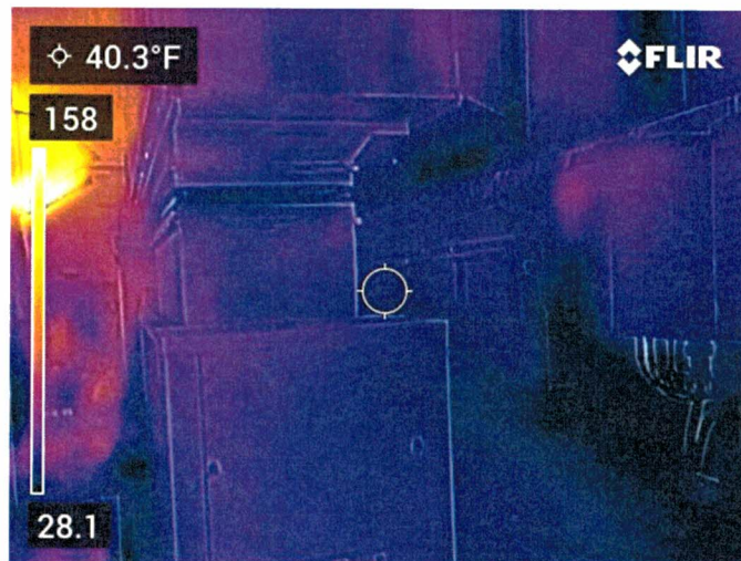
Figure 8. Thermal image of a penthouse showing warm air at top of penthouse and cold air down toward the floor of the penthouse
