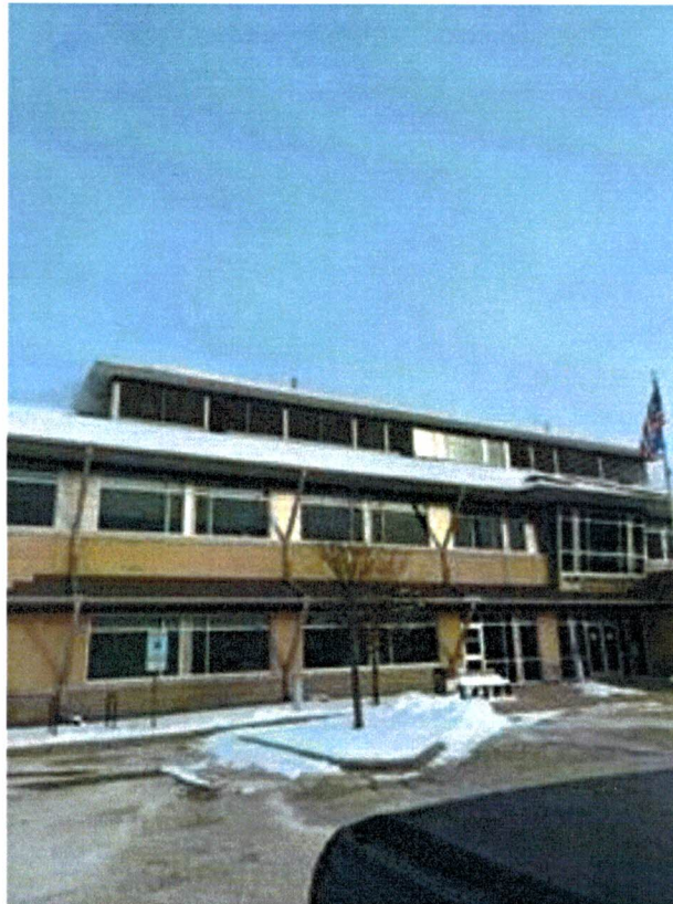
Figure 1. Exterior photo showing penthouses and intake louvers.
