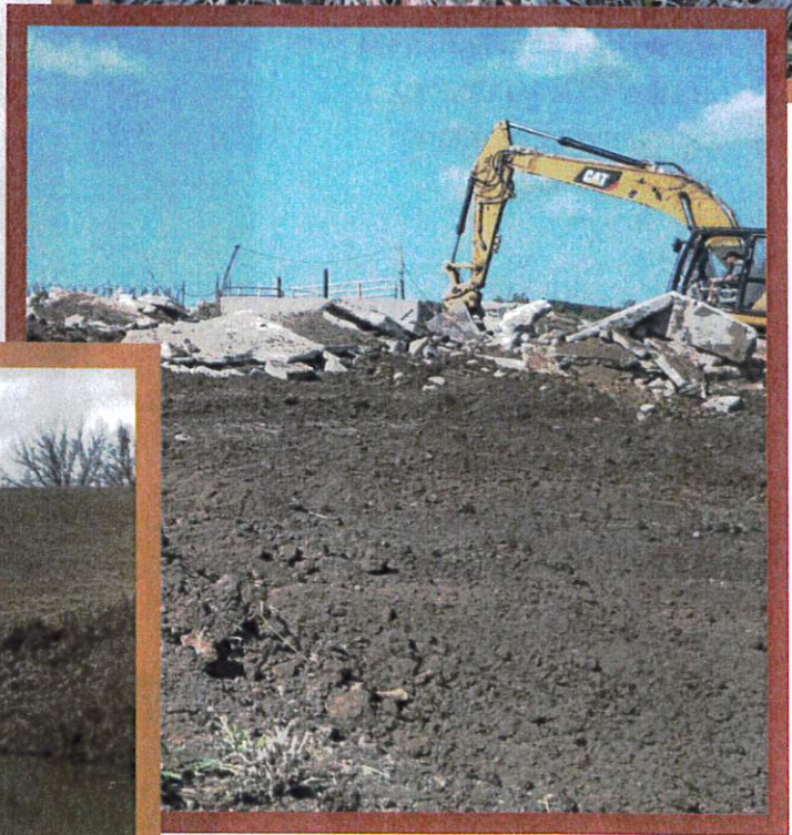
Manure storage closure in process
