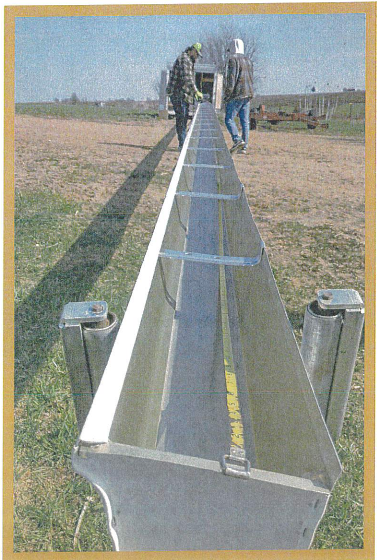
Roof gutter ready to be installed
