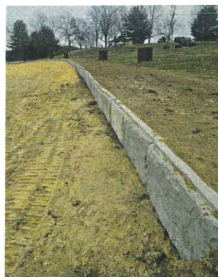
New retaining wall installed at Blackhawk Lake beach
