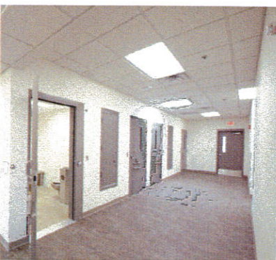
MCF-Faribault Intake & Receiving Building
