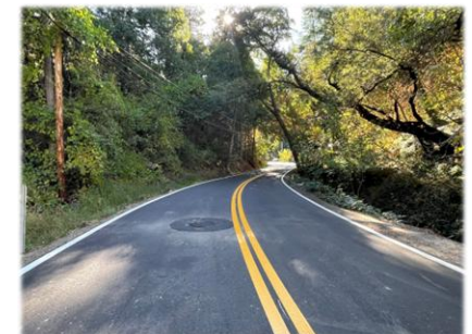
Smith Flat Road Project – New Pavement
