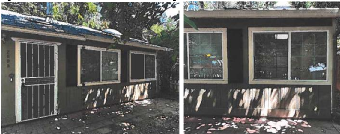
Figure 3. Picture of Western Elevation Following Work
