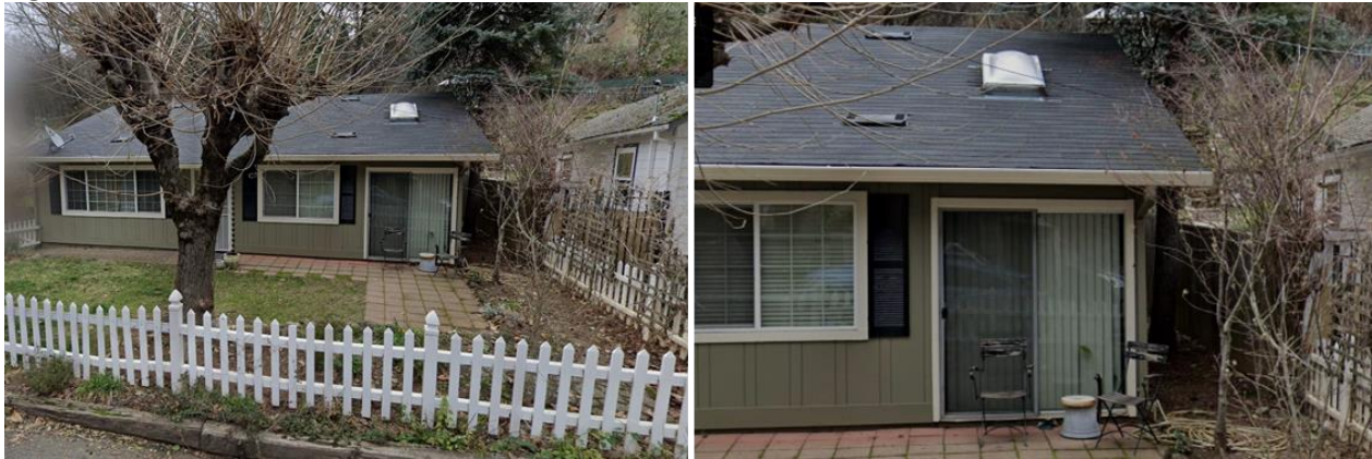
Figure 2. Picture of Western Elevation Prior to Work
