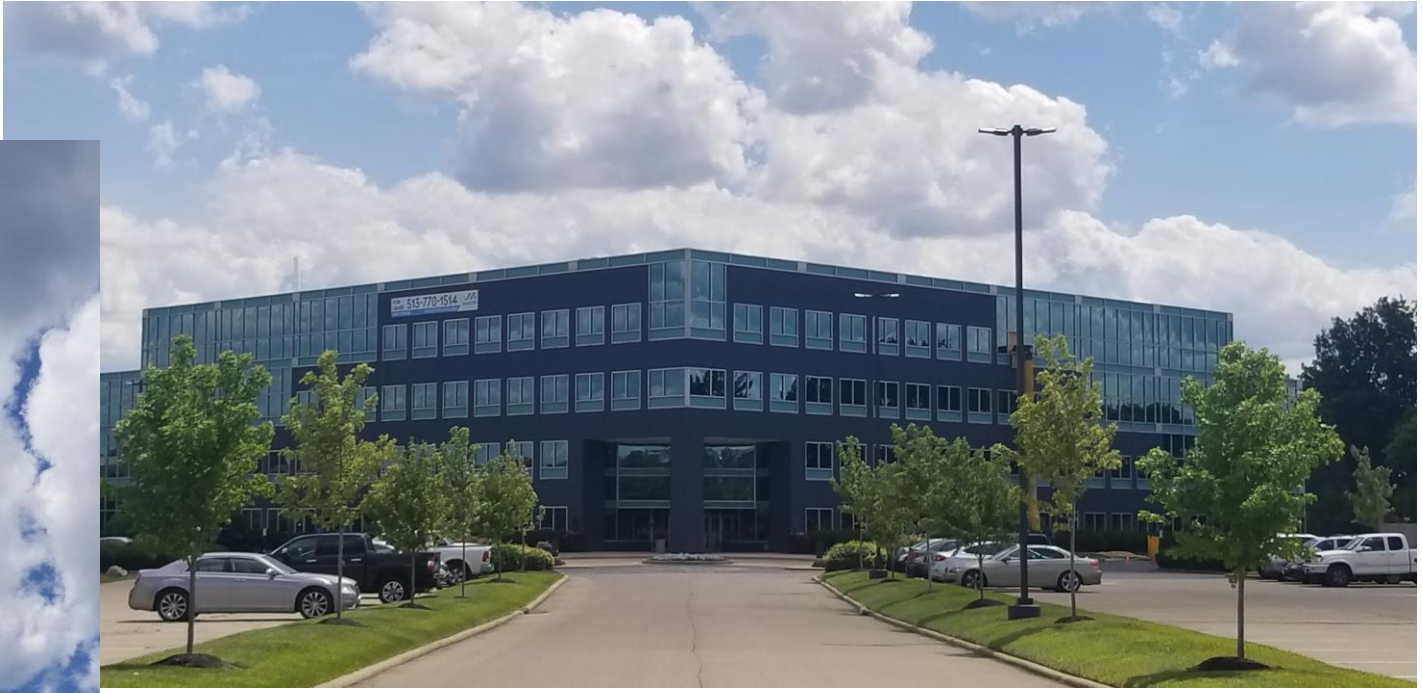
Cincinnati Ohio installation Ericsson and Commscope antennas wrapped.
