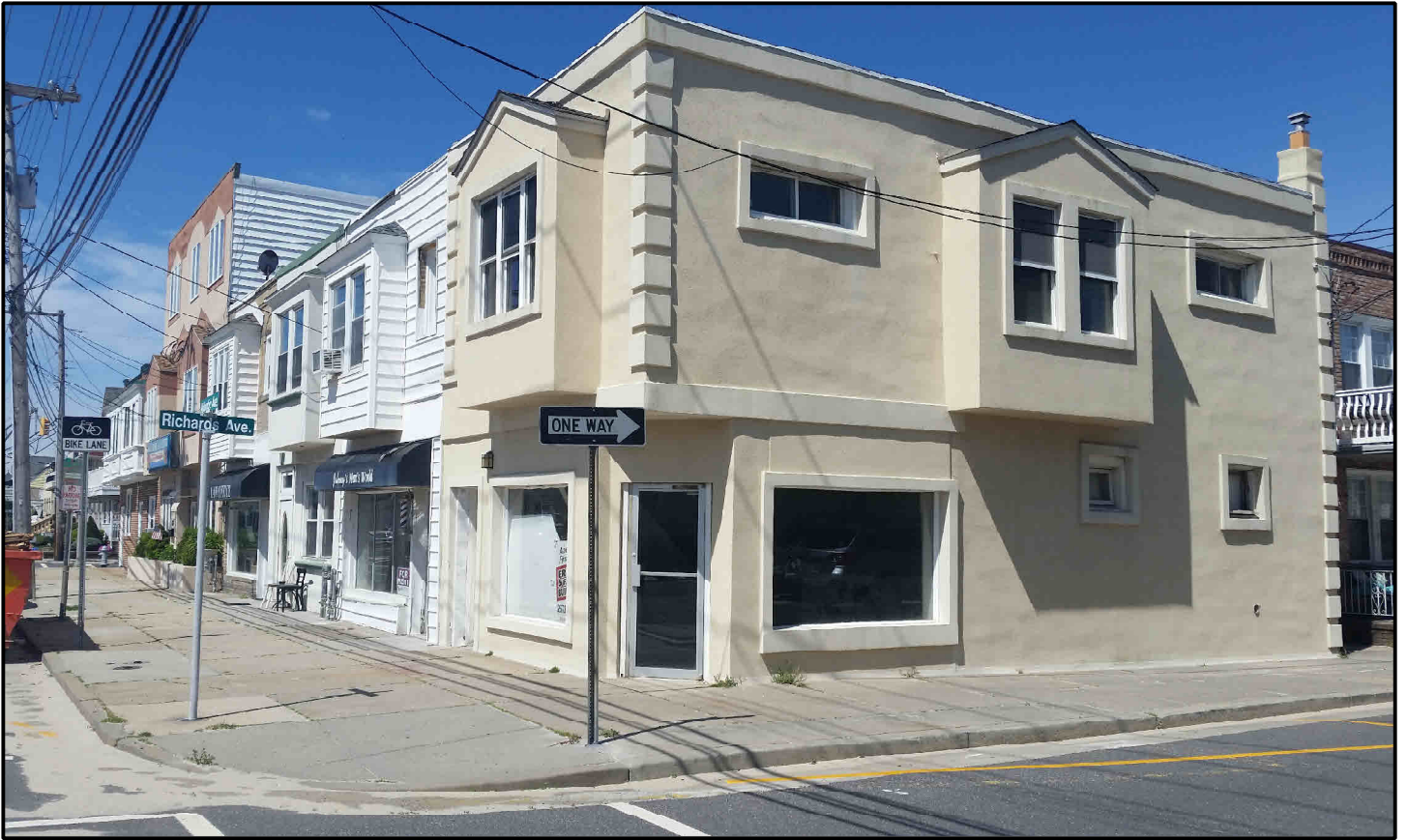
FRONT OBLIQUE VIEW
