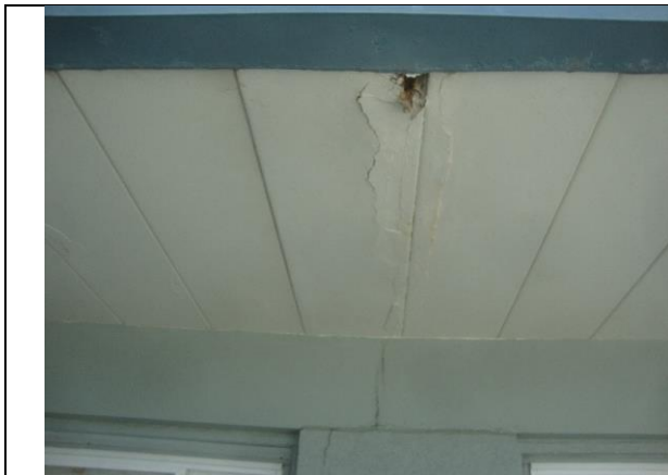
Photo #21 – Crack in second floor hollow core slab.
