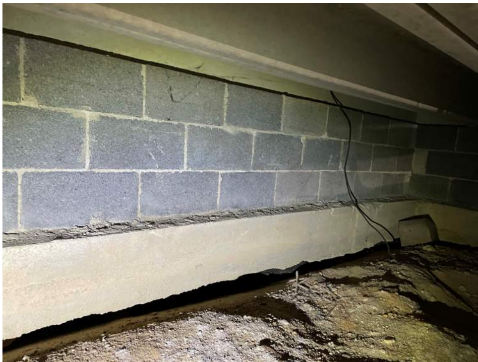
Undermining of soil beneath foundation grade beams.
