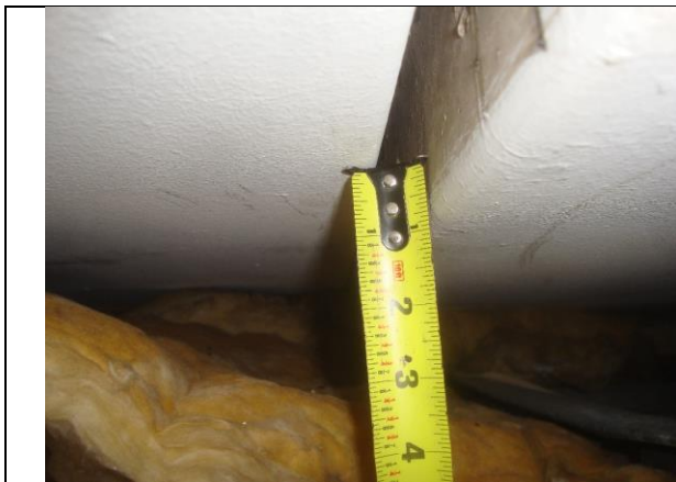
Photo #23 – Out of plane roof slabs between slabs. (Unit 24)
