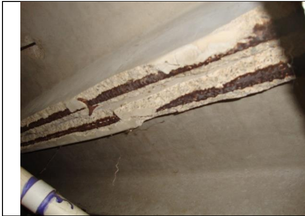
Photo #13 – Example of spalled concrete at first floor channel beams. (Building E)
