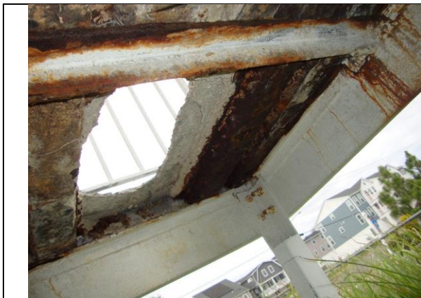
Photo #35 – Progressive deterioration of the all steel north staircase.
