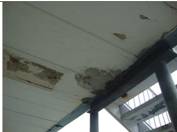
Photo #34 – Cracked slabs at upper landing with added steel shoring.
