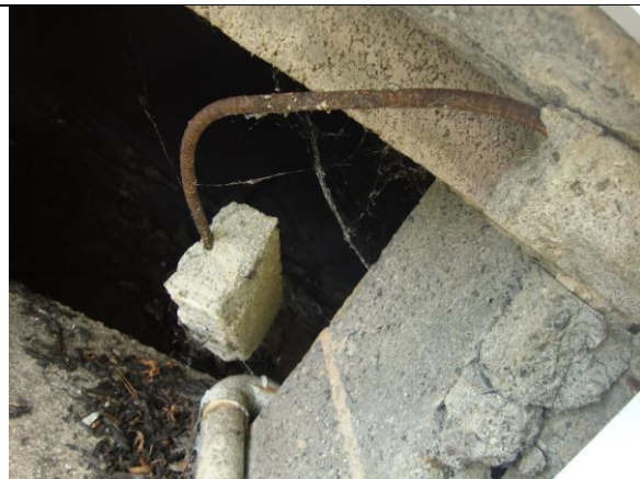
Photo #16 – Failed precast lintel at crawl space opening. (Building A)
