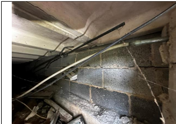
Photo #9 – Example of CMU wall displacement. (Building B)
