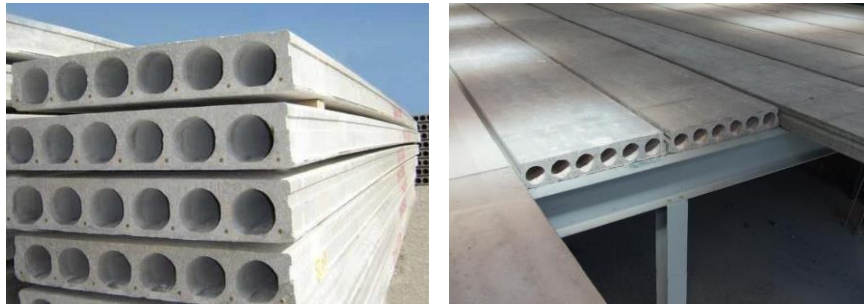
Figure #5 – Examples of Hollow Core Slabs. (Source: Structural Prestressed Industries, Inc.)
