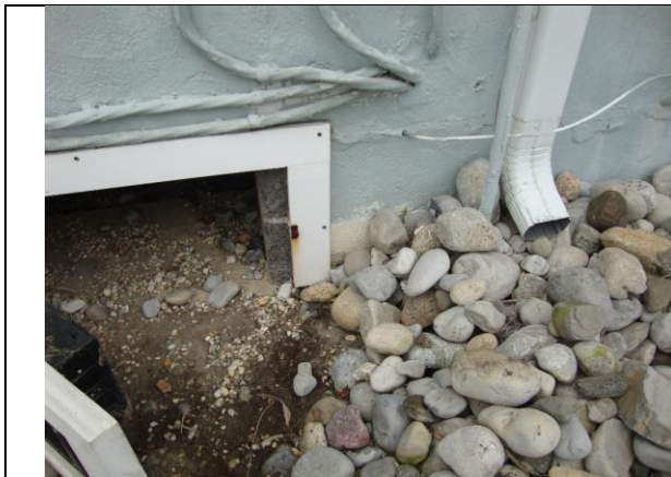
Photo #15 – Roof downspout discharging next to subgrade crawl space opening. (Building C)
