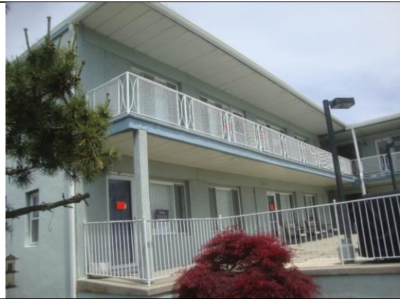
Photo #2 – Overview of cantilevered walkway balconies.
