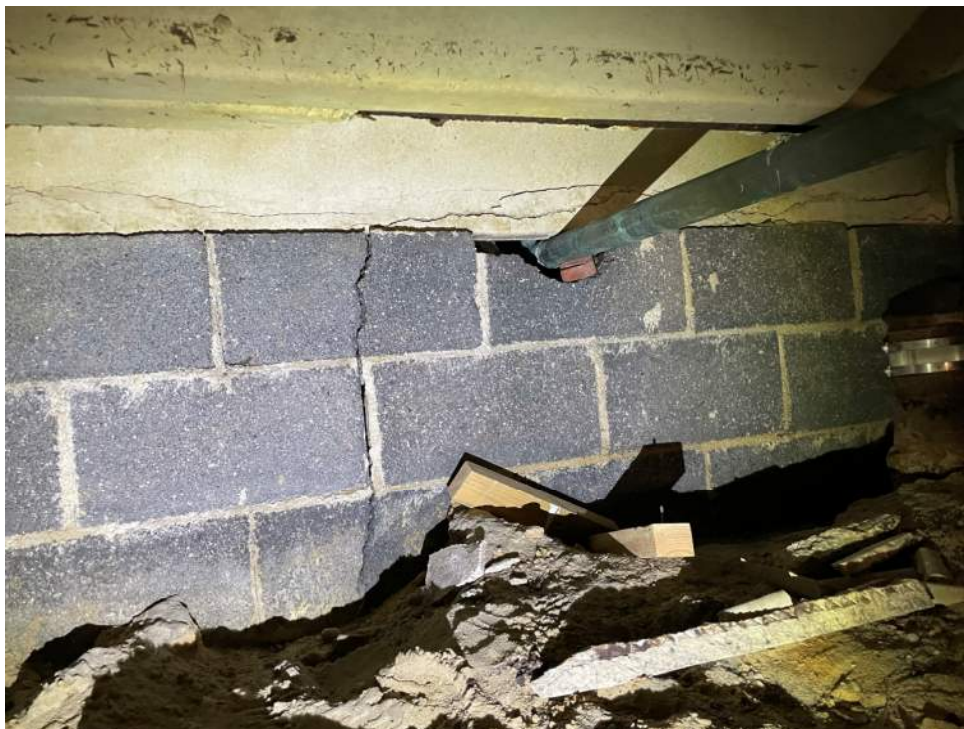
Foundation wall and grade beam failures
