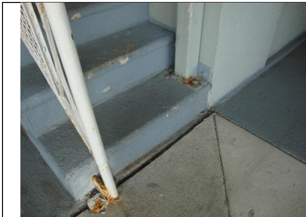
Photo #27 – Steel shoring is supported on stair step.
