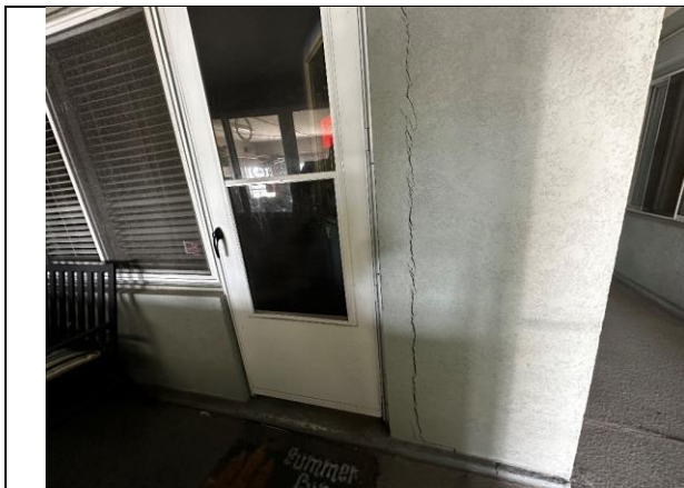
Photo #29 – Example of vertical cracks in exterior CMU walls. (Building B)
