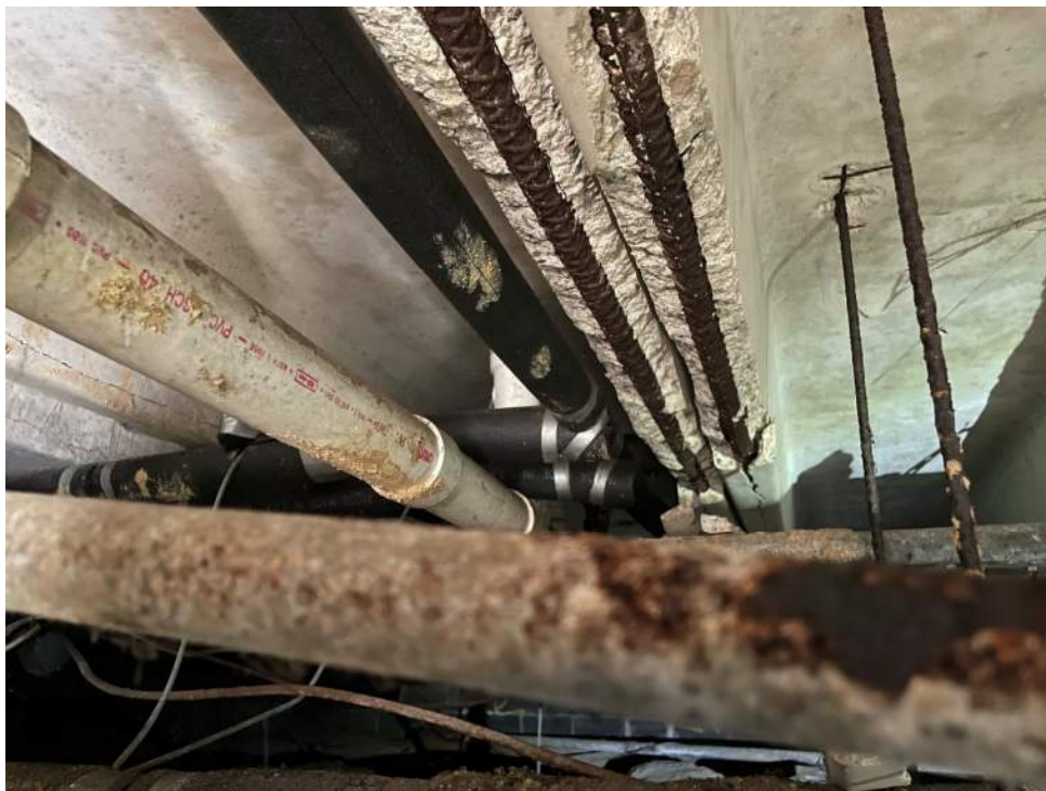
Corrosion of reinforcing and spalling of concrete in first-floor beams.
