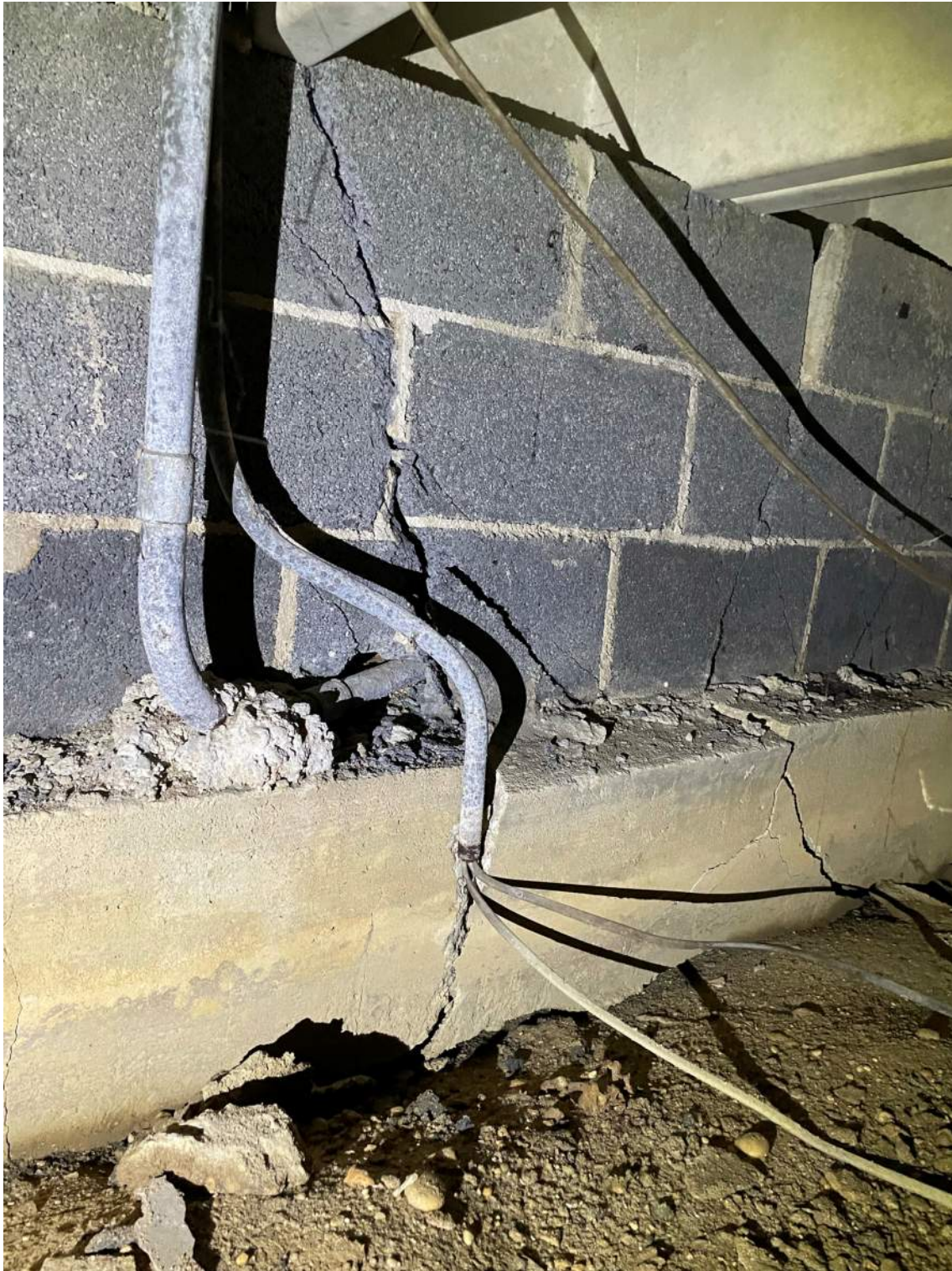
Foundation wall and grade beam failure.
