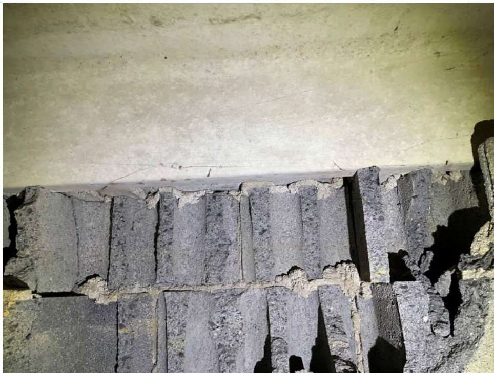
Foundation wall failures.
