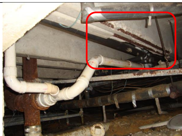
Photo #12 – Spalling of concrete cover at first floor channel reinforcing. (Building D)
