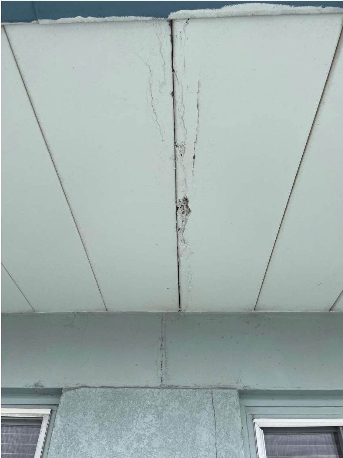
Typical corrosion-related spalling of cantilevered pre-cast planks for elevated walkway. Note cracking at lintel bearing that has developed since last painting.
