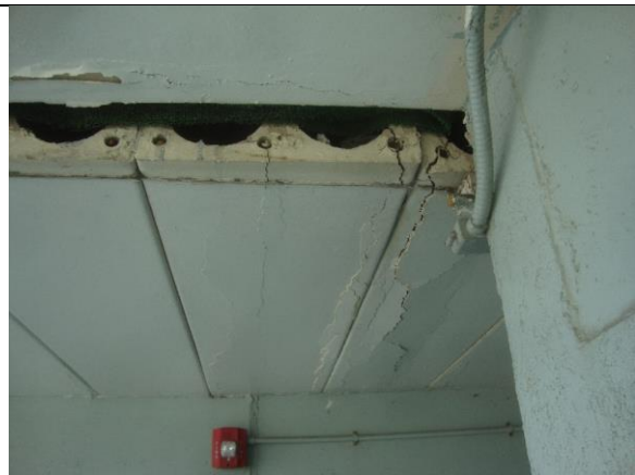
Photo #22 – Differential settlement between building sections. (Building E)
