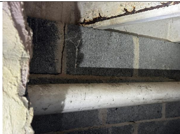
Photo #10 – Deteriorated channel at bearing wall and settlement cracks in wall. (Building B)
