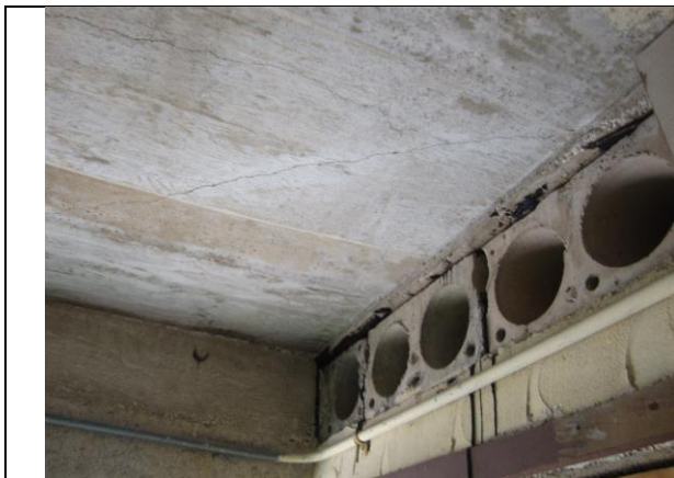
Photo #41 – Stress cracks in the roof slab of the one-story rear storage room.
