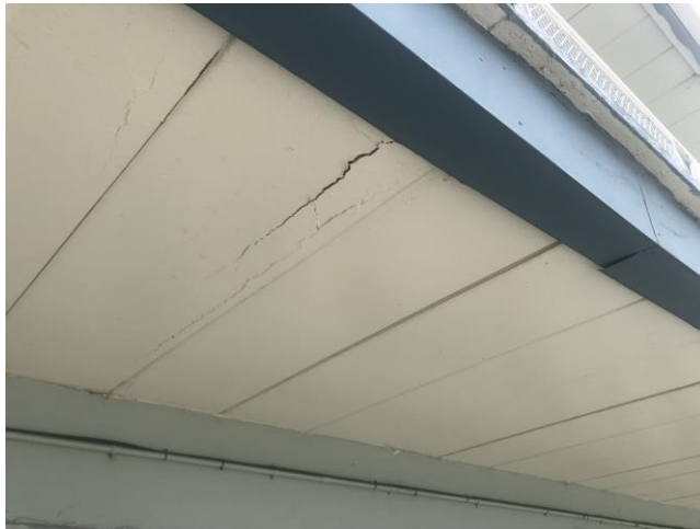
2 nd Floor walkways Note cracks with need of repairs or restoration
