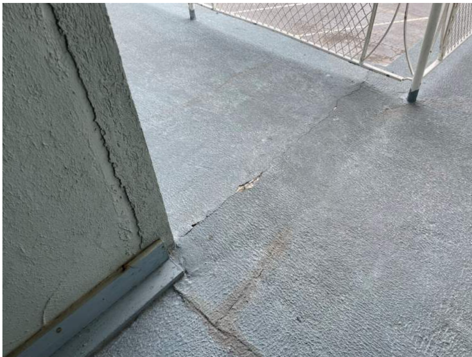
Differential settlement between modules readily visible at cantilevered walkway intersection, creating potential tripping hazard.
