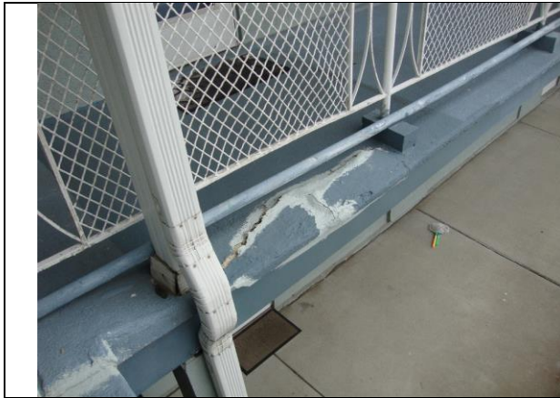
Photo #19 – Concrete spall of second floor hollow core slab. (Building D)
