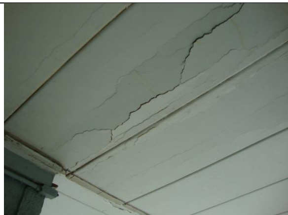
Photo #18 – Cracked second floor hollow core slab
