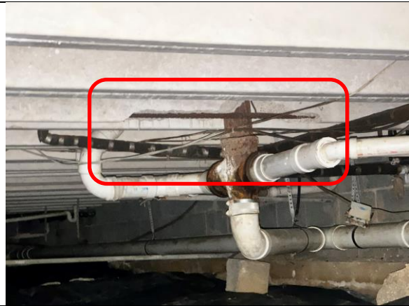
Photo #14 – Exposed and deteriorating reinforcing steel. (Building B)
