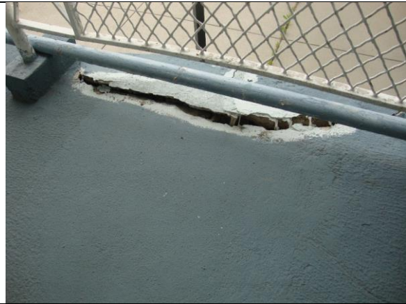
Photo #20 – Concrete spall of second floor hollow core slab. (Building D)
