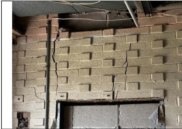
Photo #31 – Settlement cracks in non-bearing wall of the south storage room.
