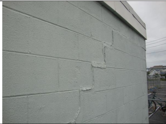
Photo #38 – Settlement crack in laundry room exterior wall.
