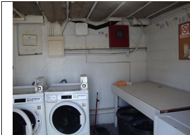
Photo #39 – Settlement crack in laundry room interior wall.
