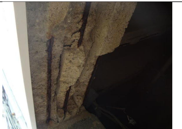
Photo #30 – Spalled precast lintel at crawl space opening. (Building E)
