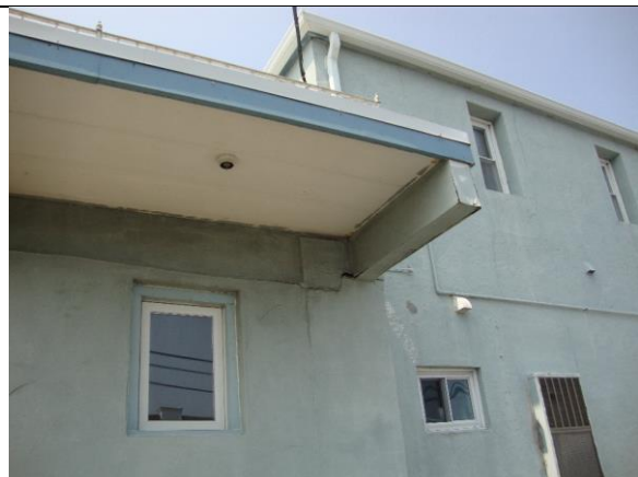
Photo #42 – Cracks at cantilevered beam at Units 15 & 31.
