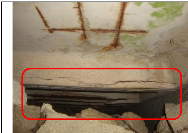
Photo #17 – Spalled concrete and rusting rebar. (Building A)
