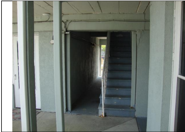
Photo #25 – South breezeway with added steel shoring for precast lintel.
