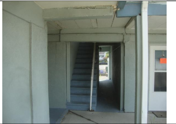
Photo #26 – North breezeway with added steel shoring for precast lintel.
