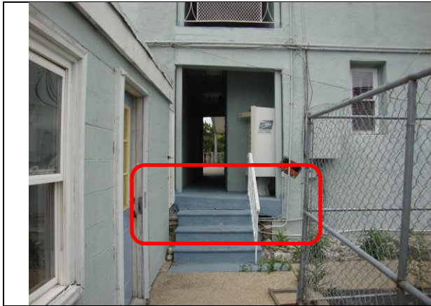
Photo #7 – Example of uneven floors due to settlement between building sections (D & E).
