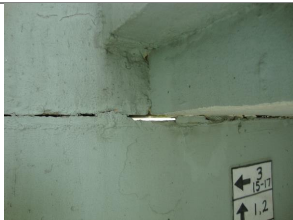
Photo #24 – Open gaps between wall and second floor due to settlement.
