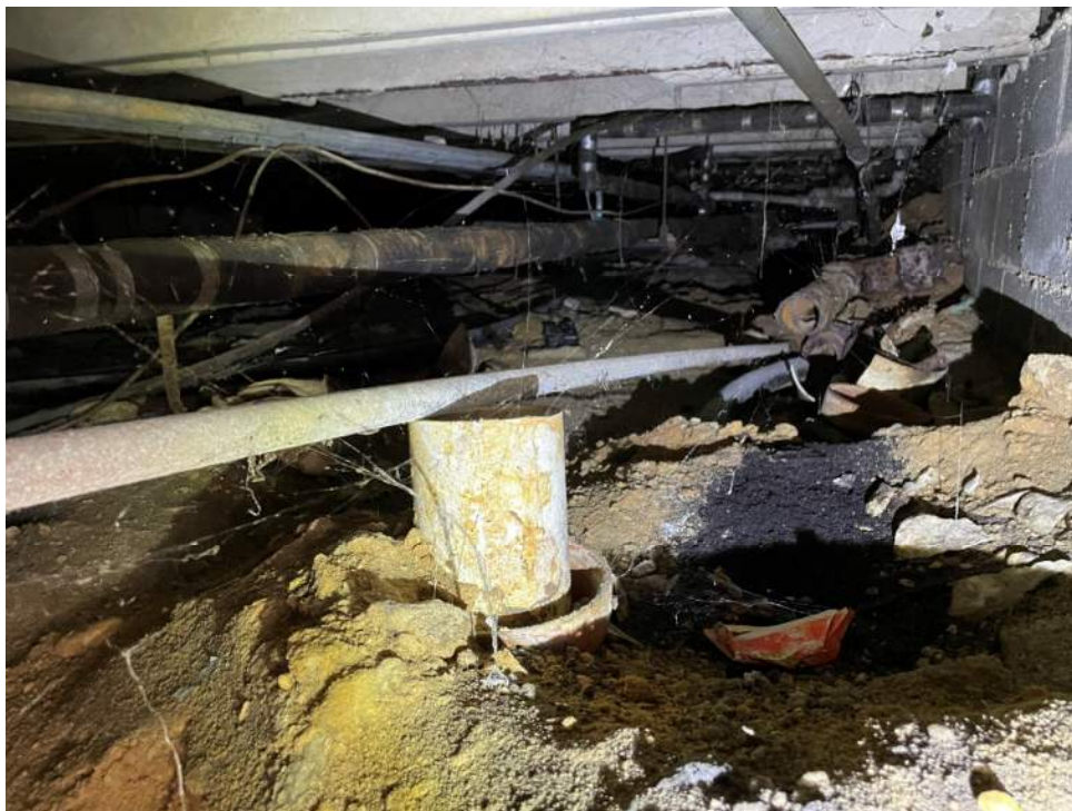
Corrosion of reinforcing and bearing support of first-floor beams. Note difficult access and obstruction of repair area by utilities.
