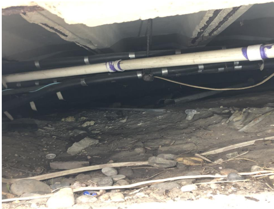
Corrosion of reinforcement and concrete spalling in first floor beam (crawlspace 1 and 2)
