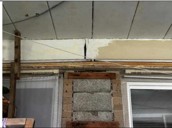
Photo #32 – Signs of settlement in the south storage room.
