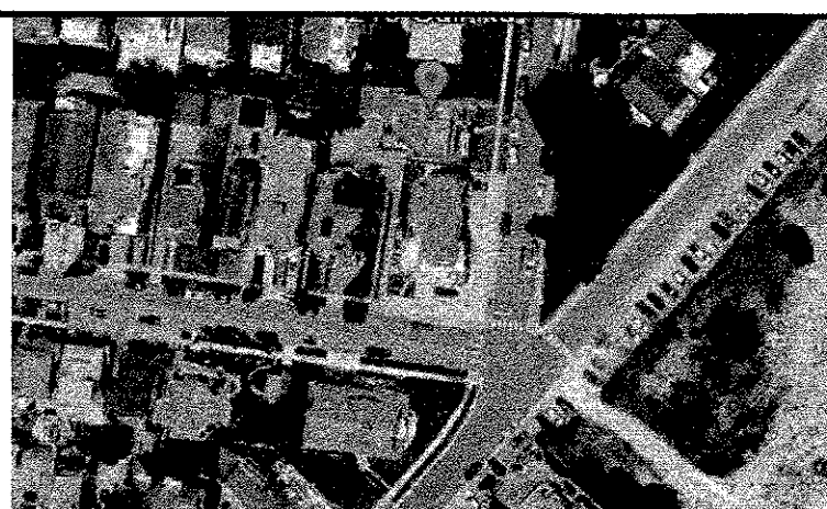
3 AERIAL VIEW N.T.S. - FOR REFERENCE ONLY COURTESY OF GOOGLE EARTH
