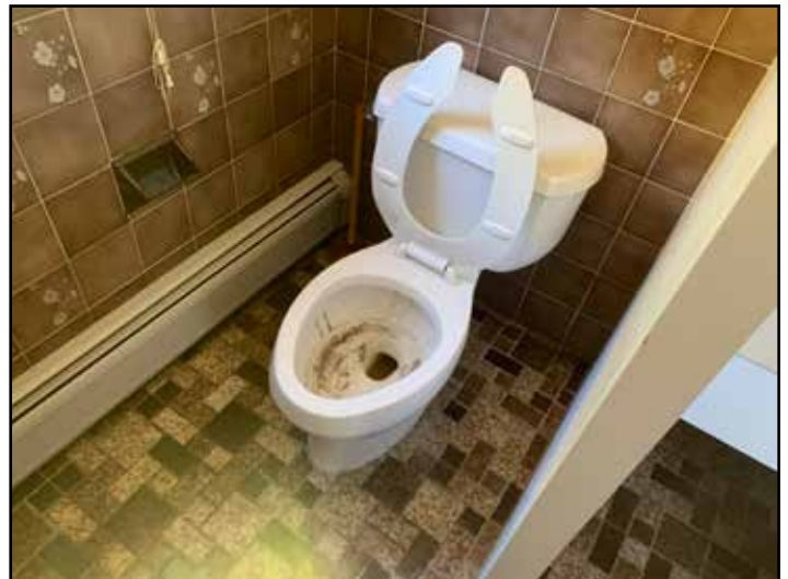
Image 15: Existing vacant former day care bathroom.
