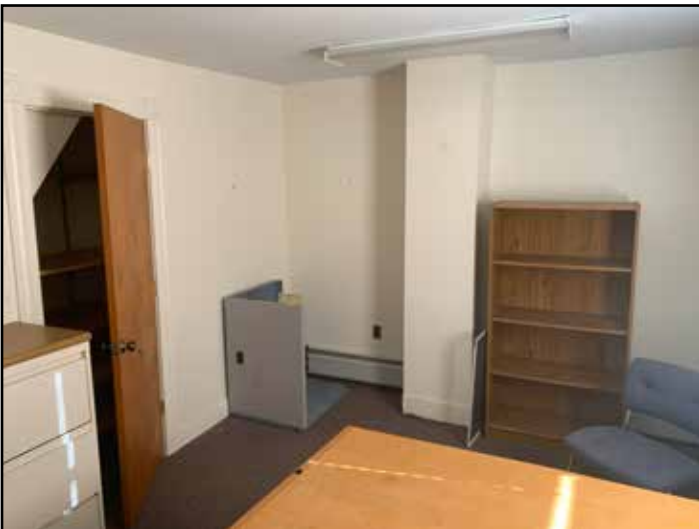
Image 14: Existing vacant former day care interior room.
