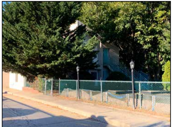
Image 51: View of damaged fencing along former playground area.
