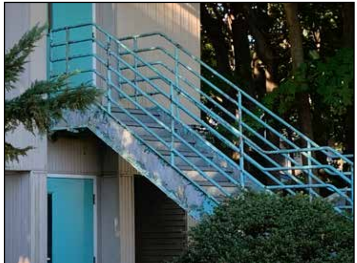
Image 49: View of stairs (egress) from second level of the second building.
