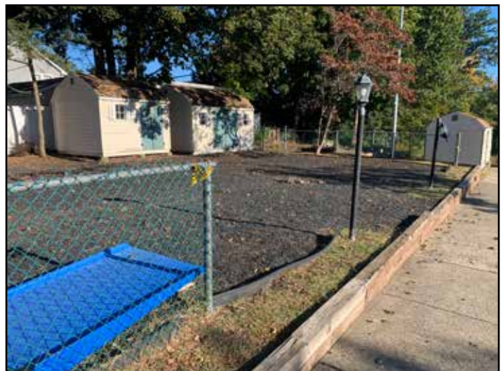
Image 57: View of damaged formering playground area with missing fence.
