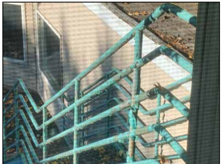
Image 39: View of metal stairs (egrees) from second floor to the former playground area.
