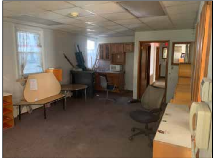
Image 11: Existing vacant former day care interior room.
