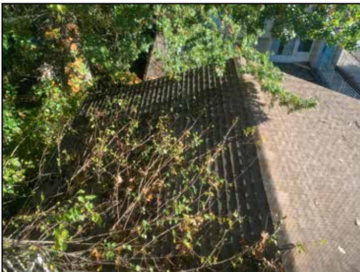
Image 18: Roof of one story portion of the former day care.
