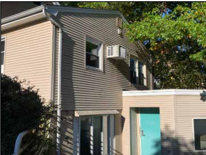
Image 44: View of side of the building facing north.
