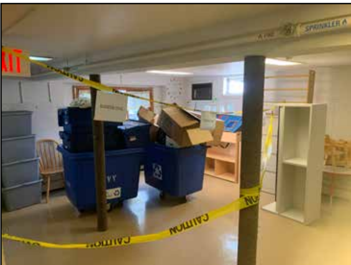
Image 24: Former classroom area.
