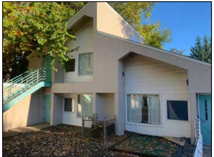
Image 45: View of side of the building facing south.
