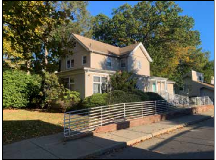
Image 1: Former day care building closest to Kingsland Street
