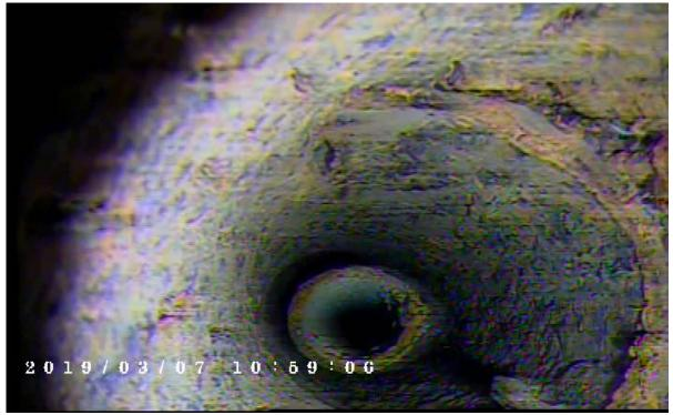
Lateral 5 - Sand-line and offest at 28 feet from valve face.
