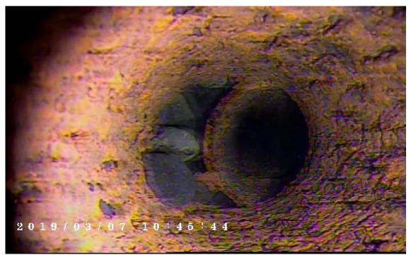
Lateral 8 - Break and cobbles at 5 feet from valve face
