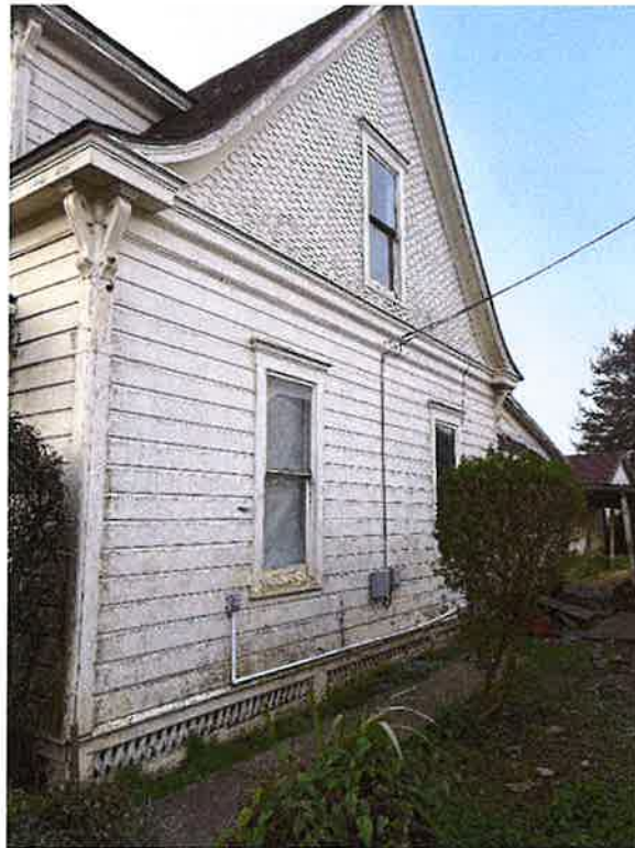
Figure 12 – North Exterior of the Original House
