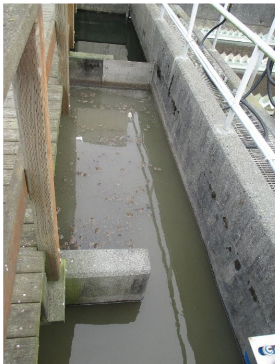
Figure 5-3. Channel to Membrane Bioreactor in Need of Baffle
