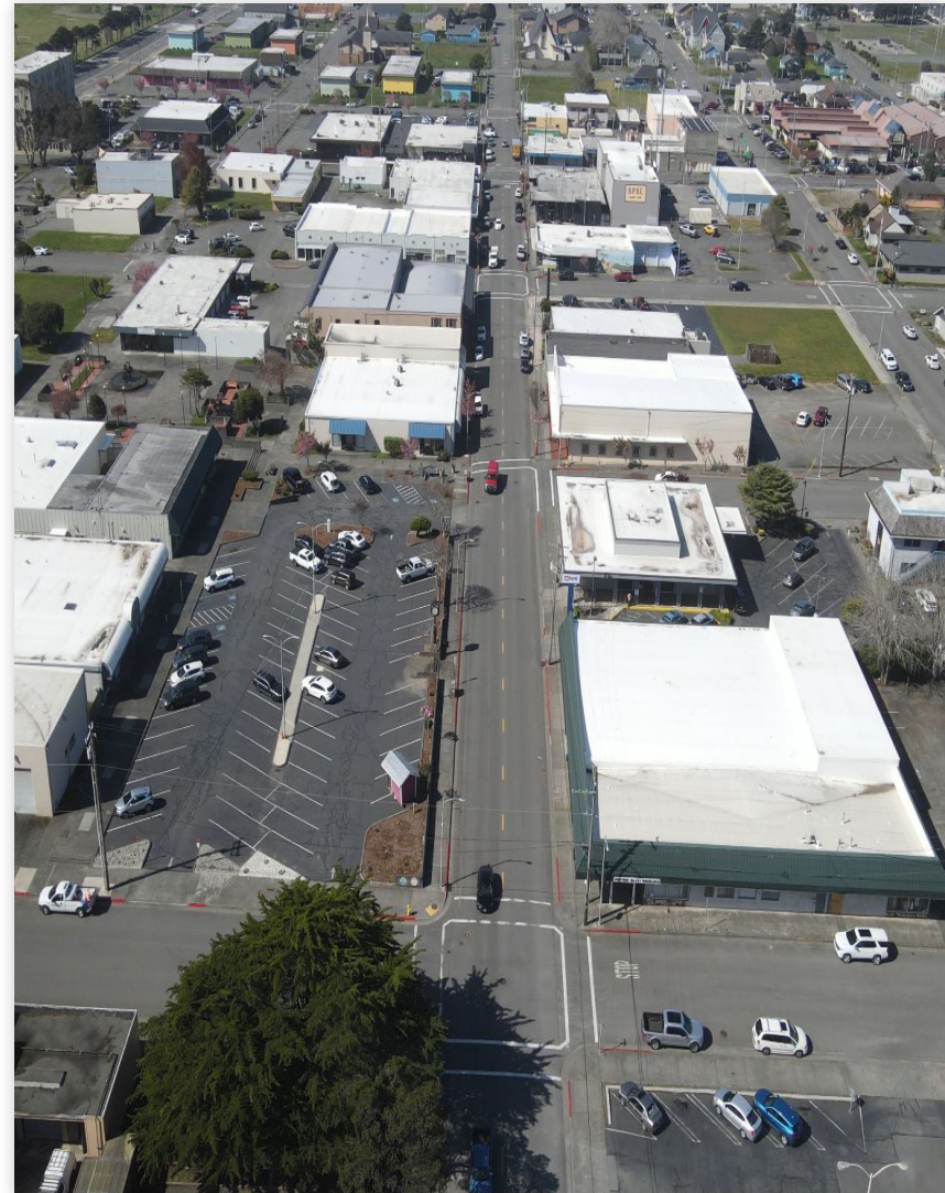
Figure 12. Downtown Third Street Looking Southwest
