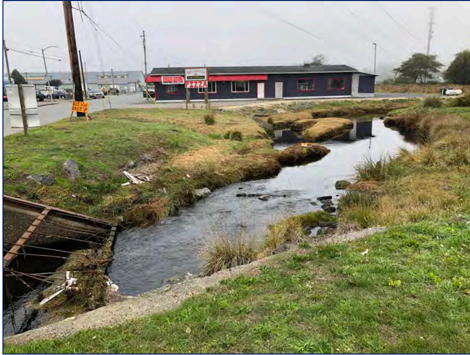
Figure 2-8. Elk Creek upstream of Hwy 101 crossing. Culvert inlet headwalls and trash rack in bottom left. Roughened channel in center. View looking upstream.
