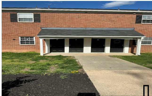
115 Willis Rd Suite E, Com- mercial Renovation, Maple- ton Square Apartments
