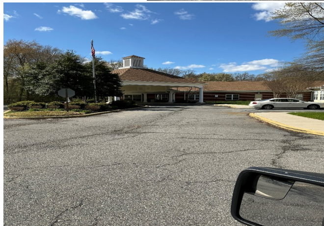
1225 Walker Rd -Commercial Renovation Cadia Rehabilitation Capitol
