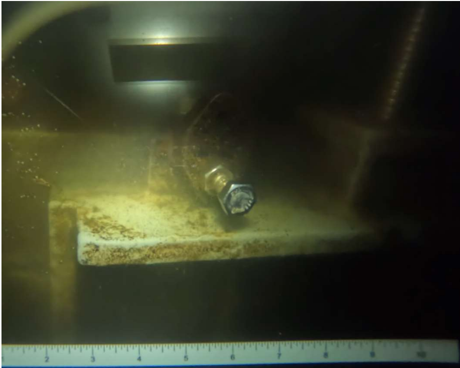
PHOTO 13: Top wedge, left side of gate
