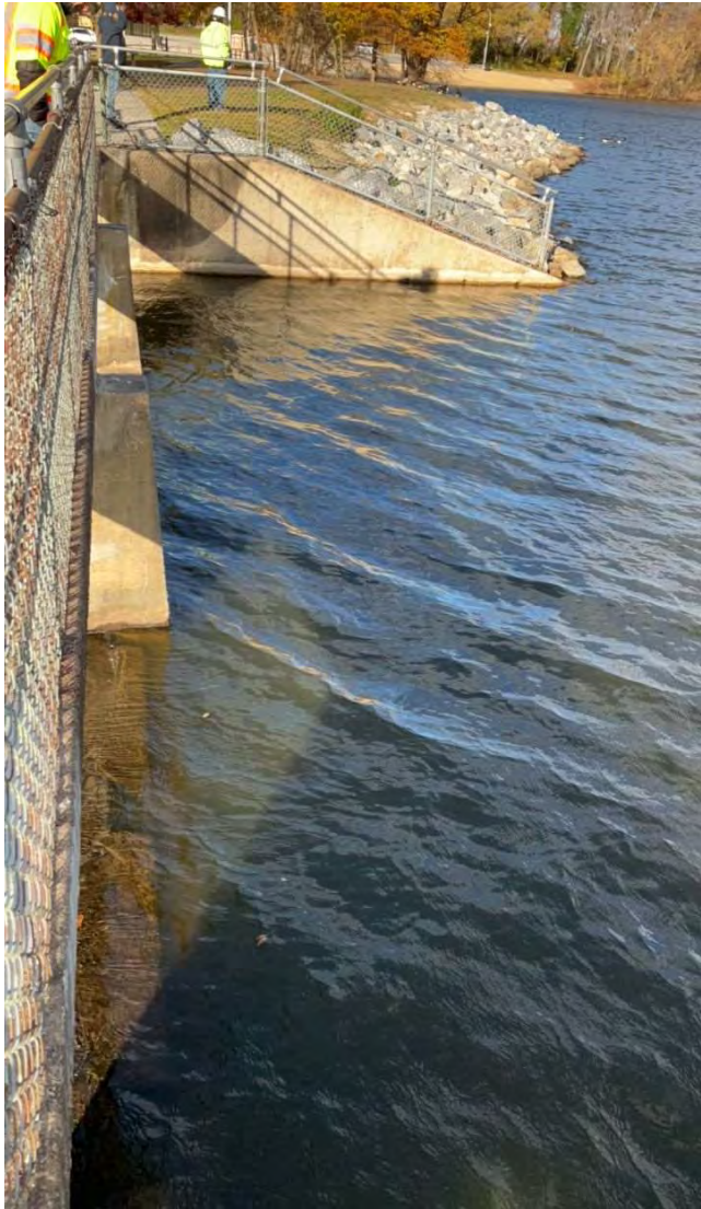
PHOTO 31: Spillway entrance channel and crest; right spillway wingwall/training wall upstream of spillway.
