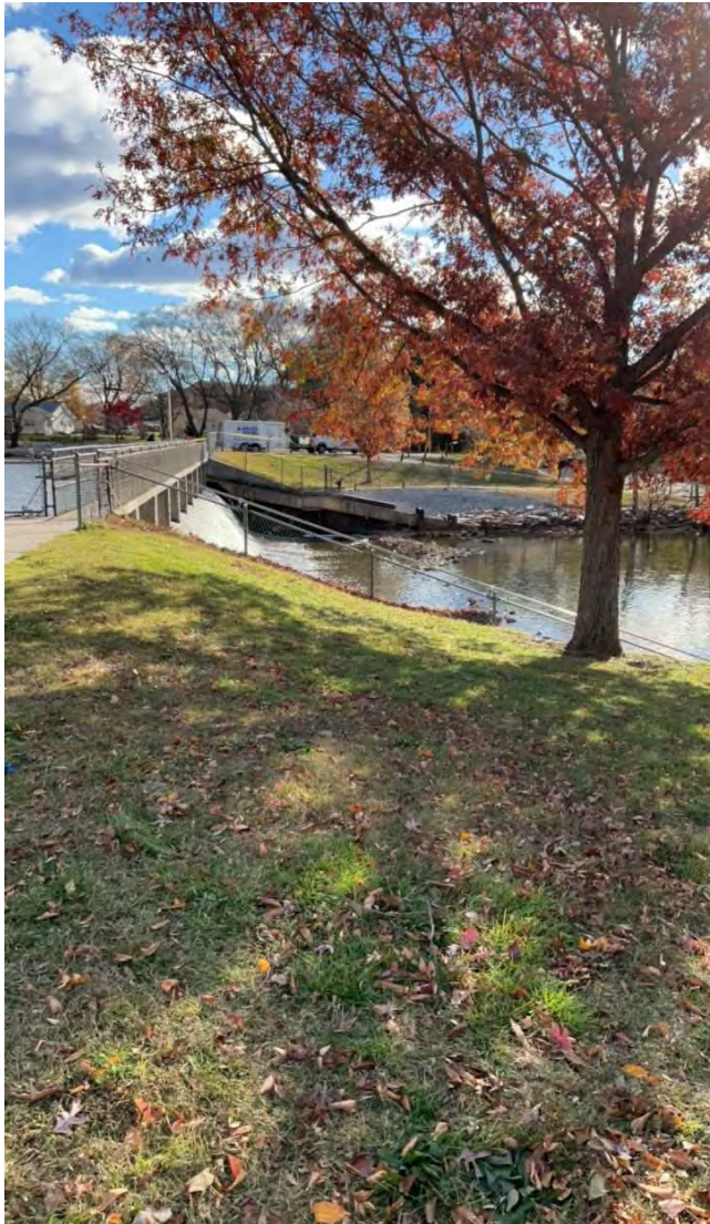
PHOTO 21: Right embankment downstream slope. Note tree adjacent to right spillway wingwall/training wall.
