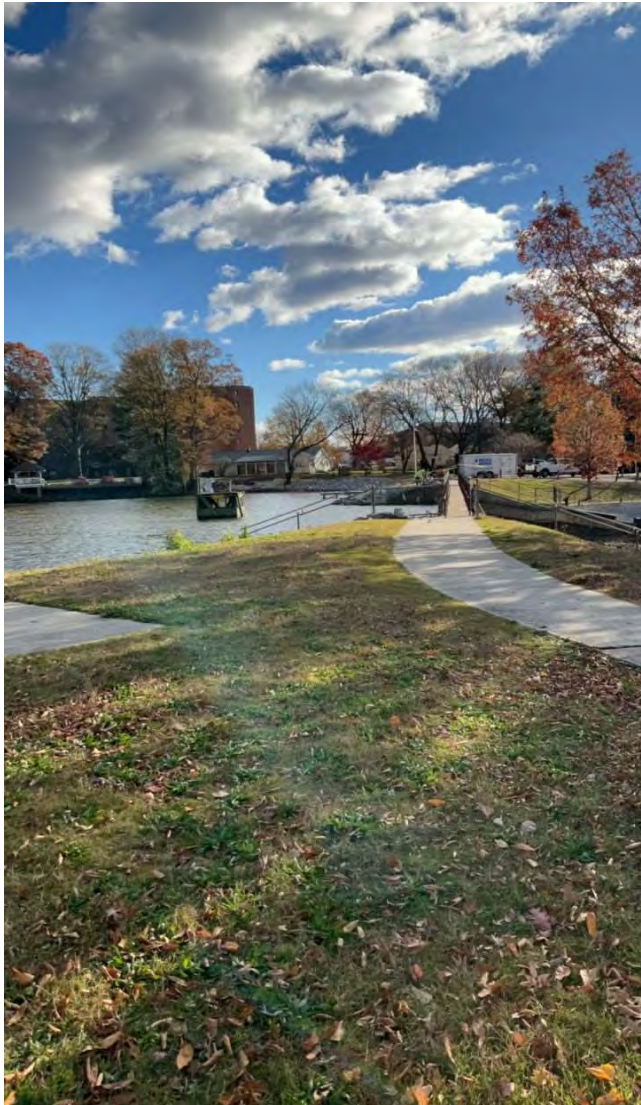
PHOTO 19: Right embankment crest, looking east.
