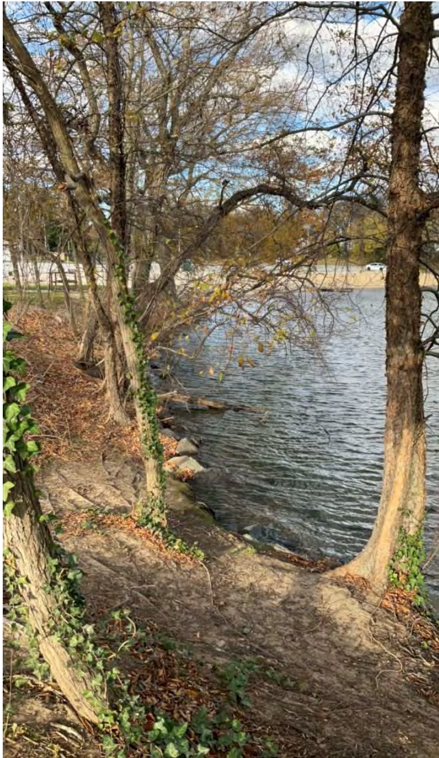
PHOTO 17: Right embankment upstream slope, west of riprap armoring
