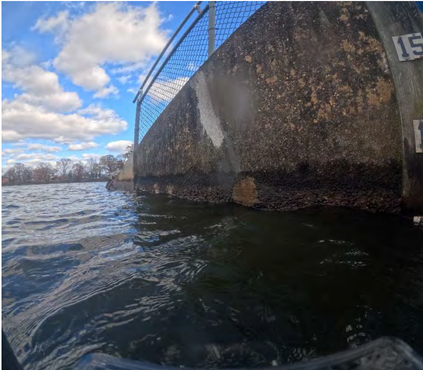
PHOTO 15: Left training wall upstream of fish ladder and spillway
