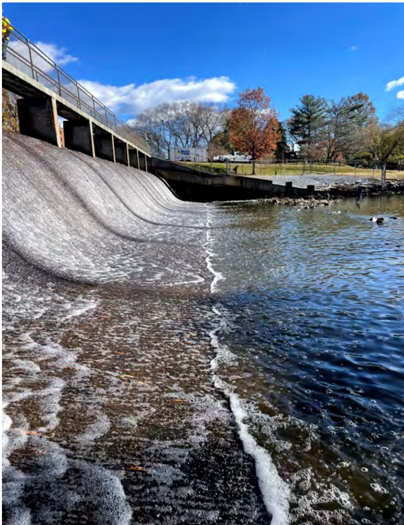
PHOTO 43: Downstream spillway apron.
