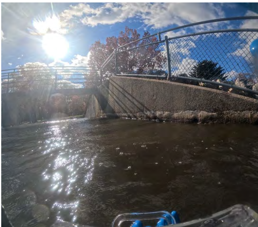
PHOTO 22: Right training wall upstream of spillway.
