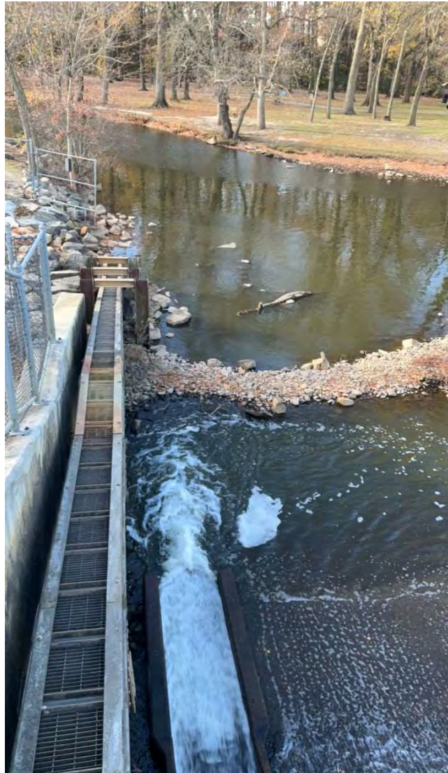
PHOTO 26: Left spillway training wall, fish ladder and low-flow chute downstream of spillway.
