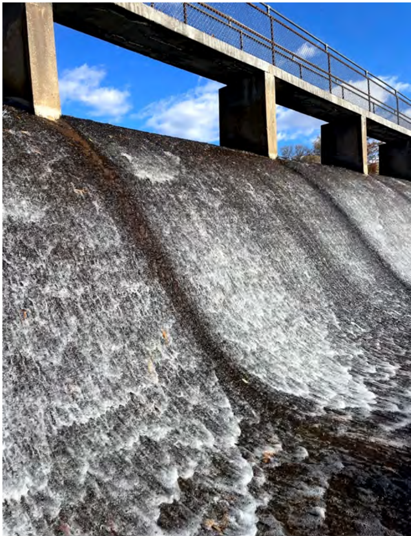
PHOTO 42: Downstream spillway face.
