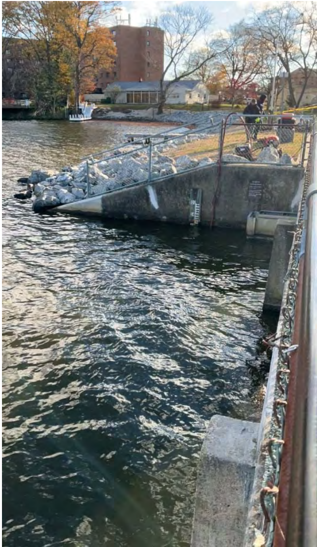
PHOTO 25: Left spillway wingwall/training wall, upstream of spillway.
