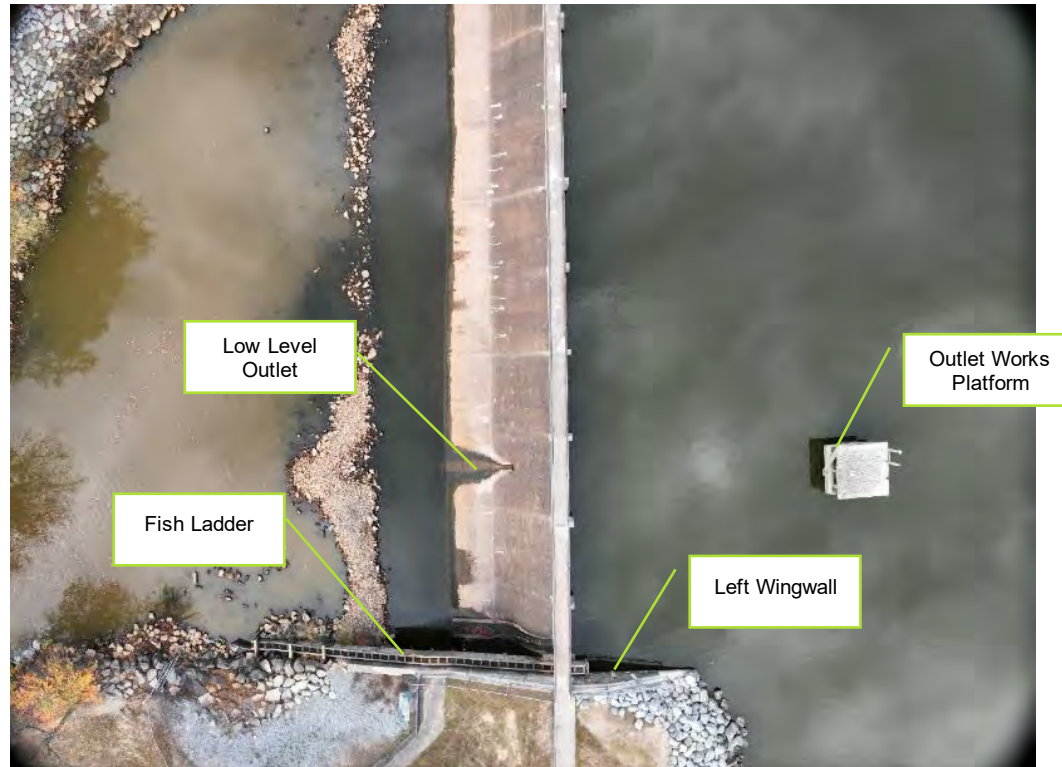
Figure 4: 2024 Aerial Photograph of Spillway and Fish Ladder
