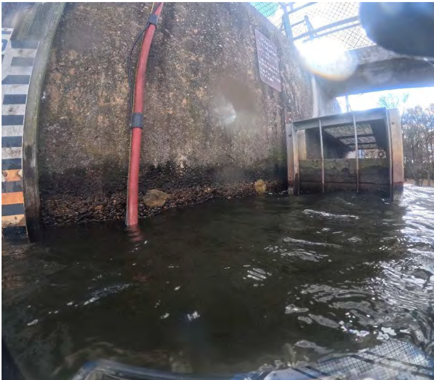
PHOTO 16: Left training wall upstream of fish ladder
