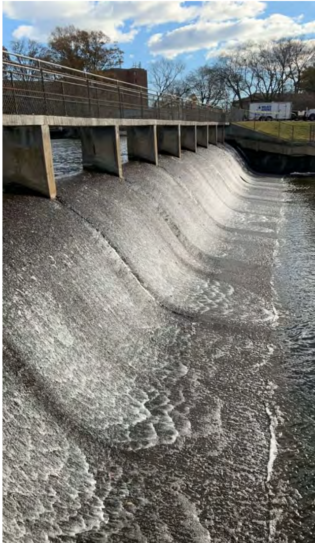
PHOTO 40: Downstream face of spillway from right side.
