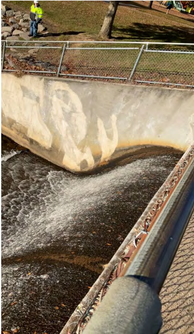
PHOTO 33: Right spillway wingwall/training wall downstream of spillway crest.
