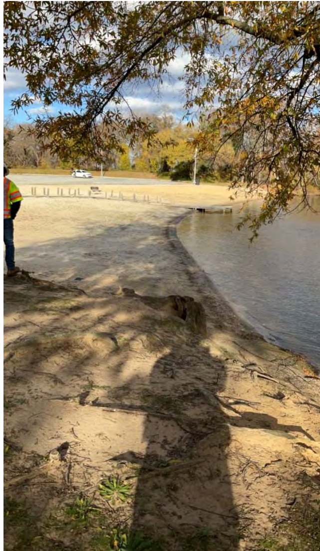
PHOTO 18: Right embankment end at public beach area.
