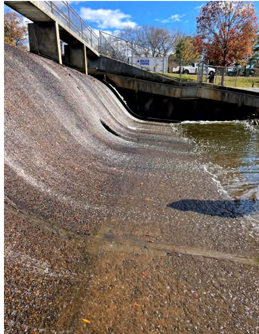
PHOTO 50: Downstream face of spillway and transition to apron. Low level outlet works discharges through spillway face.
