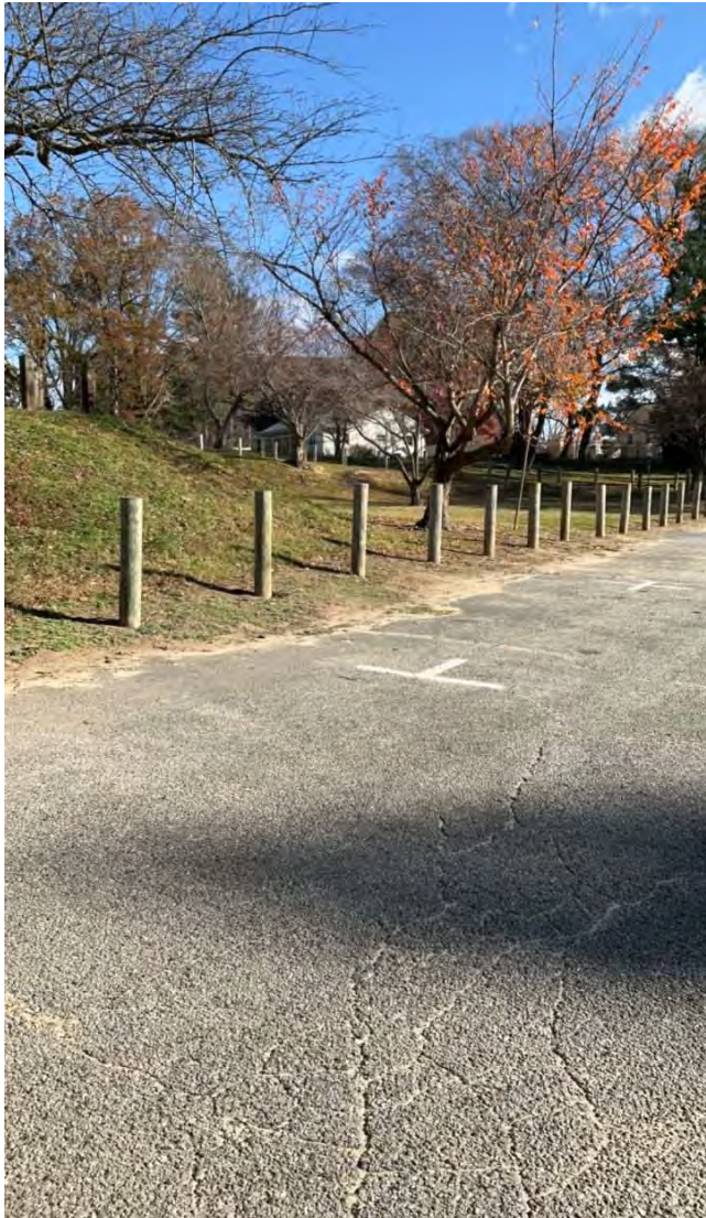
PHOTO 11: Downstream slope of left embankment above paved parking lot.
