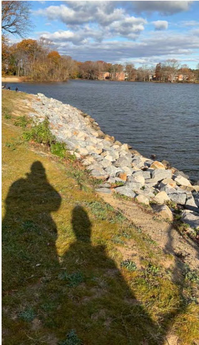
PHOTO 12: Right embankment upstream slope, looking west.
