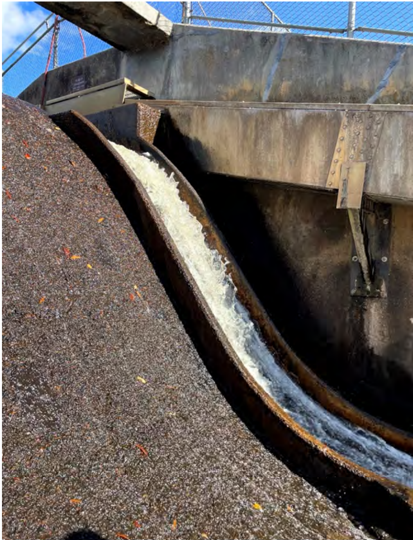
PHOTO 53: Low flow chute on downstream face of spillway at left training wall.
