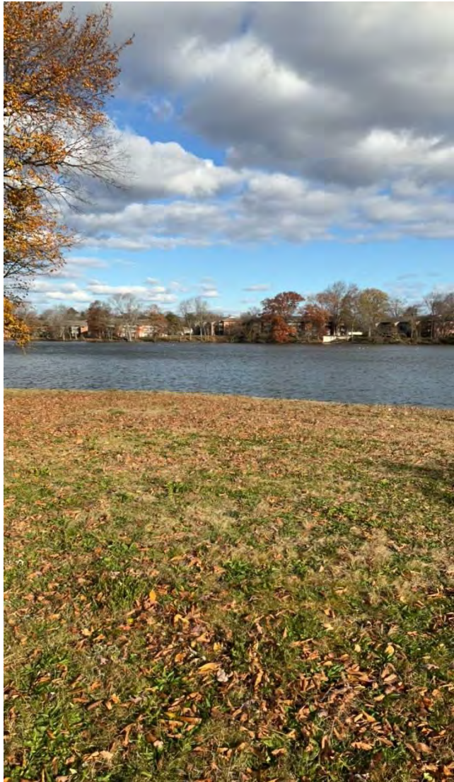
PHOTO 20: Right embankment crest and reservoir beyond.
