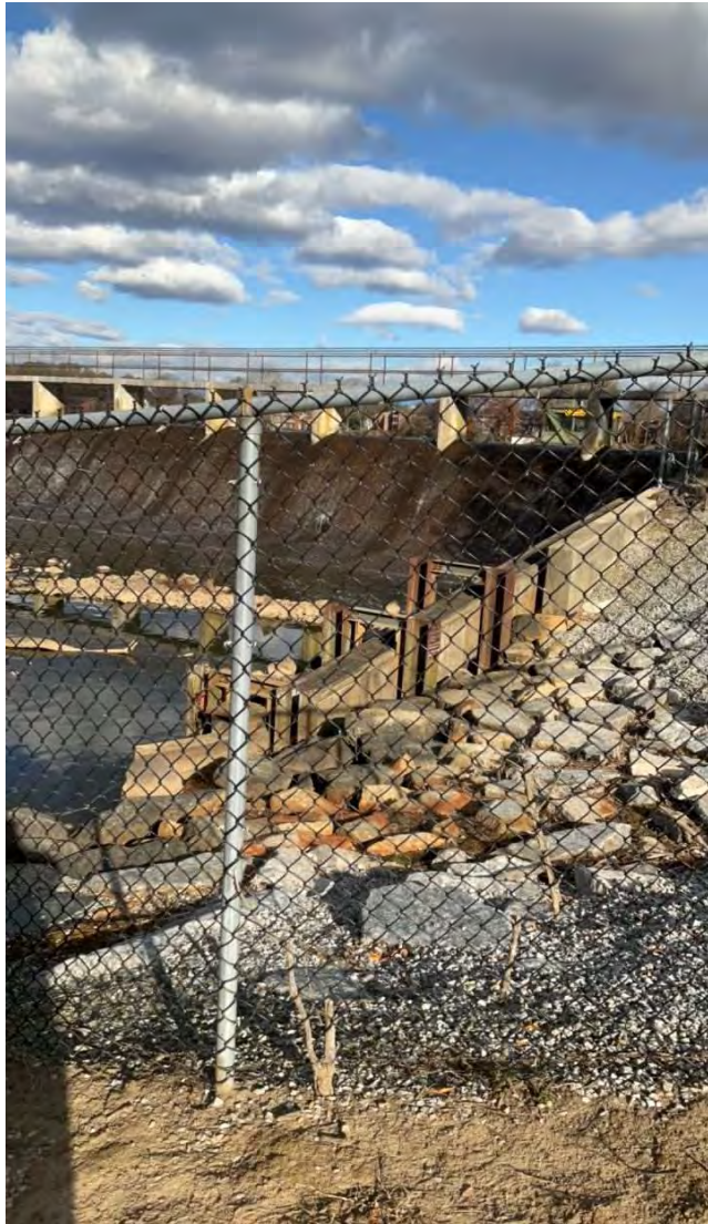
PHOTO 28: Downstream end of fish ladder on left side of spillway.
