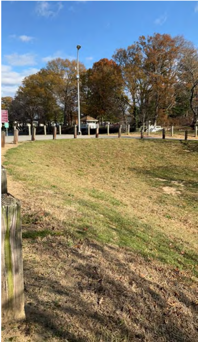
PHOTO 9: Downstream slope of left embankment.
