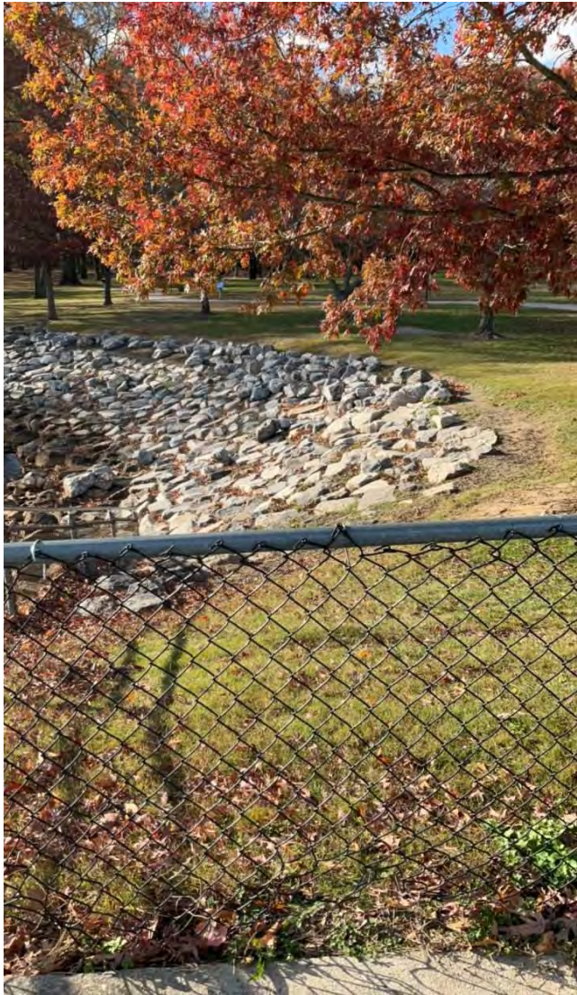
PHOTO 23: Right embankment downstream slope and riprap armoring at stilling basin and downstream channel.
