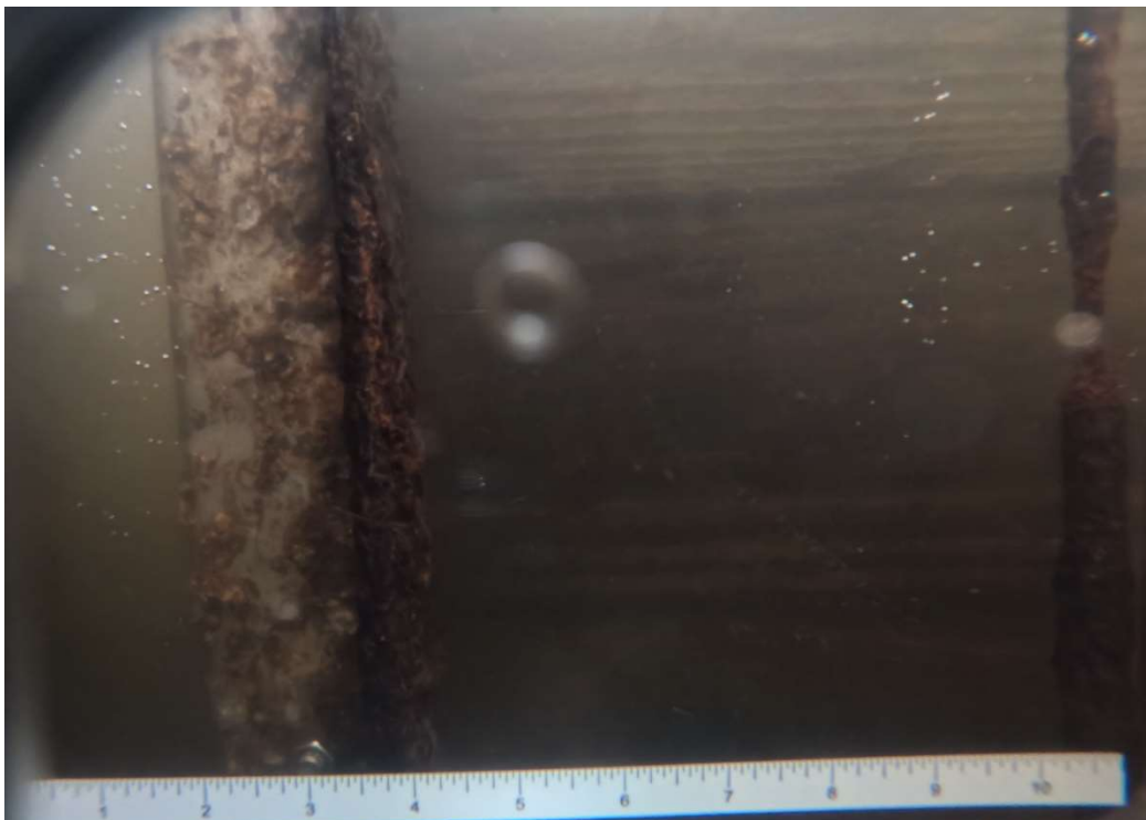
PHOTO 21: Fish ladder stop log guide below waterline
