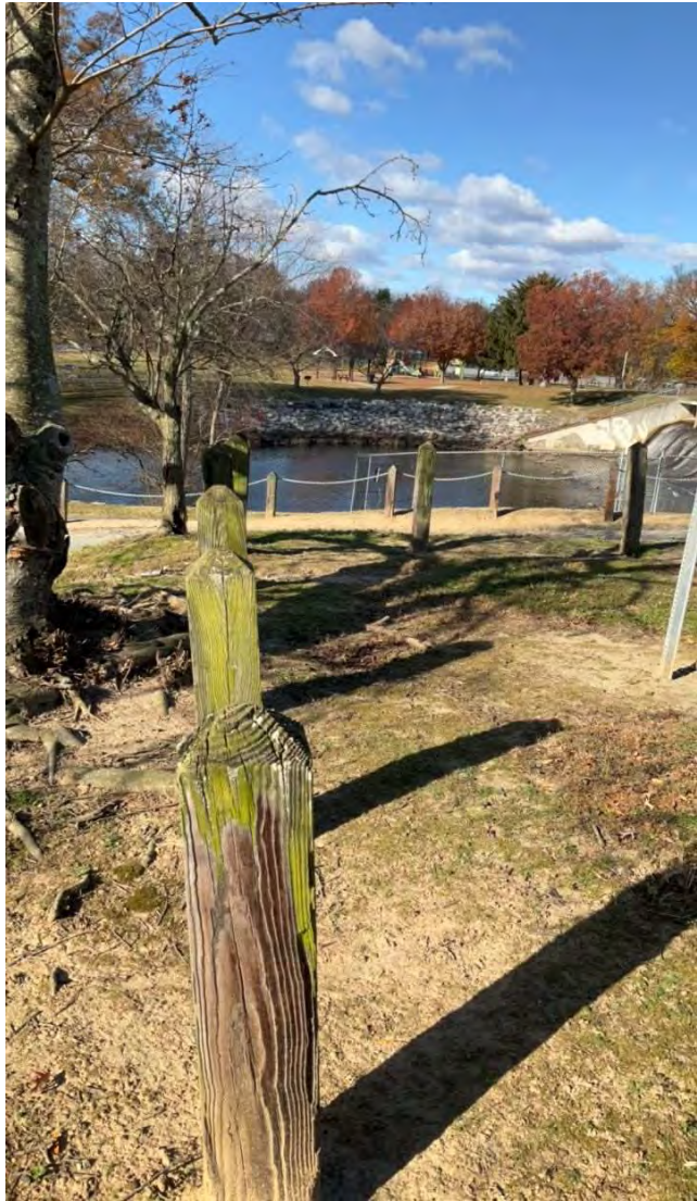
PHOTO 10: Downstream slope of left embankment above paved parking lot.
