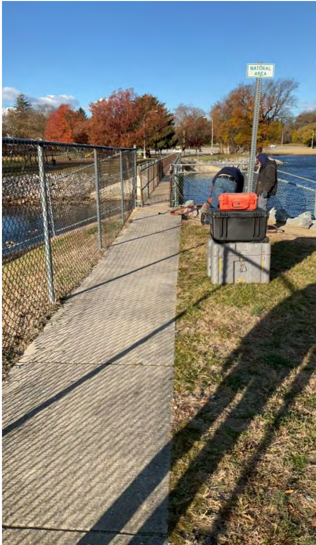
PHOTO 7: Crest of left embankment, looking west approaching spillway and pedestrian bridge.
