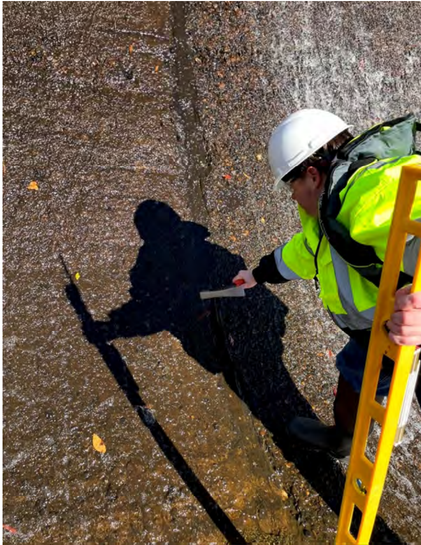
PHOTO 46: Sounding downstream face of spillway.
