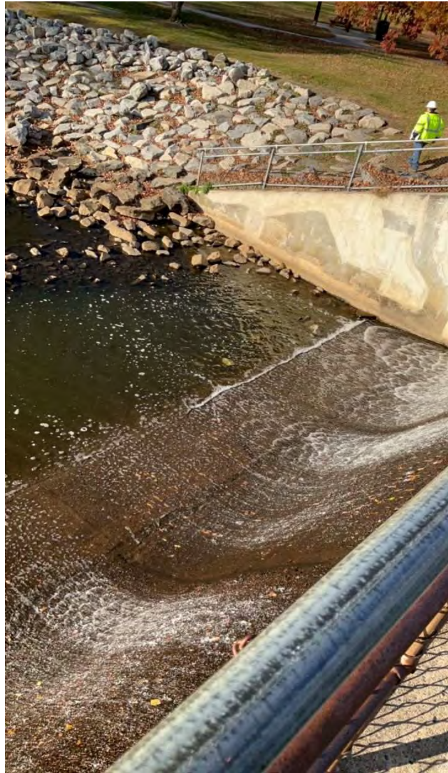
PHOTO 34: Right spillway wingwall/training wall downstream of spillway crest.
