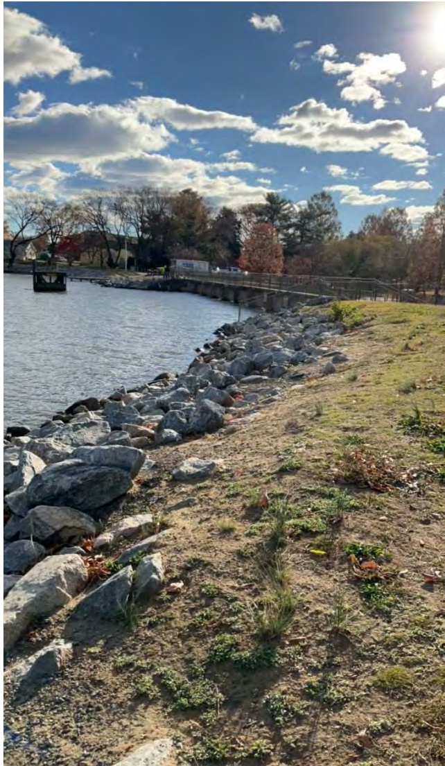
PHOTO 16: Right embankment upstream slope.
