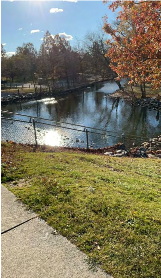
PHOTO 22: Right embankment downstream slope at right wingwall/training wall.
