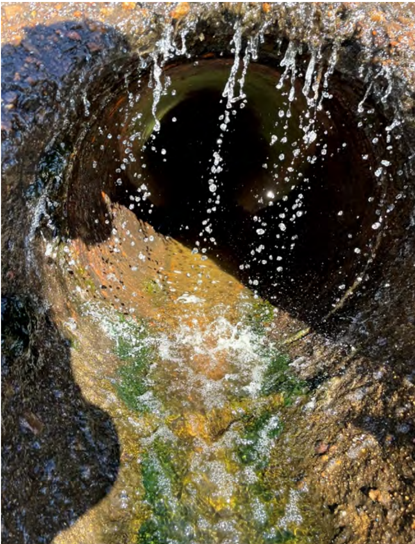
PHOTO 52: Interior of low level outlet culvert from downstream end.
