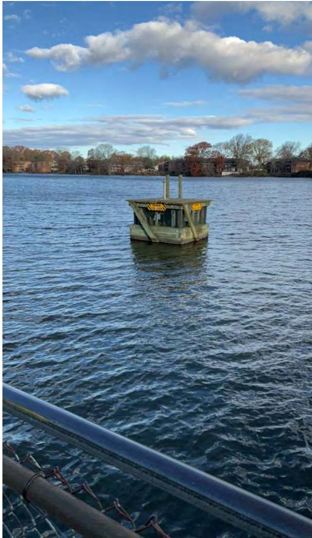
PHOTO 24: Outlet works platform located in reservoir upstream of principal spillway.
