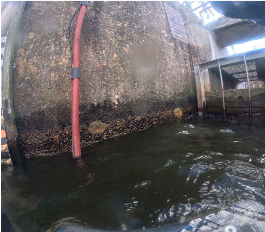
PHOTO 17: Left training wall upstream of fish ladder
