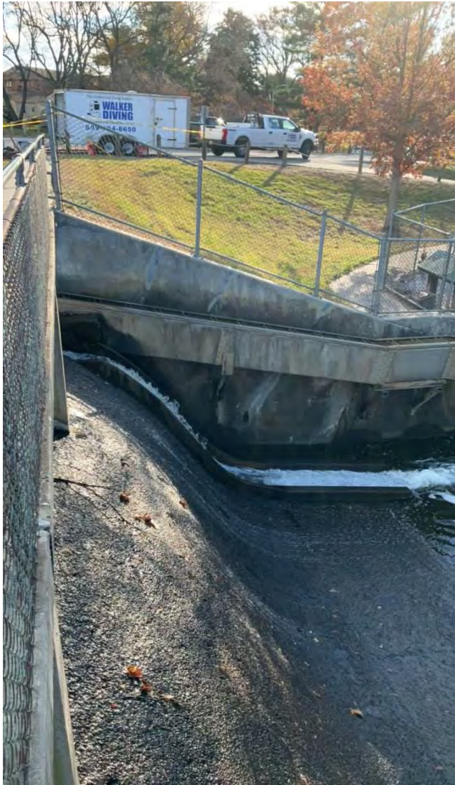
PHOTO 27: Left spillway training wall, fish ladder and low-flow chute downstream of spillway.
