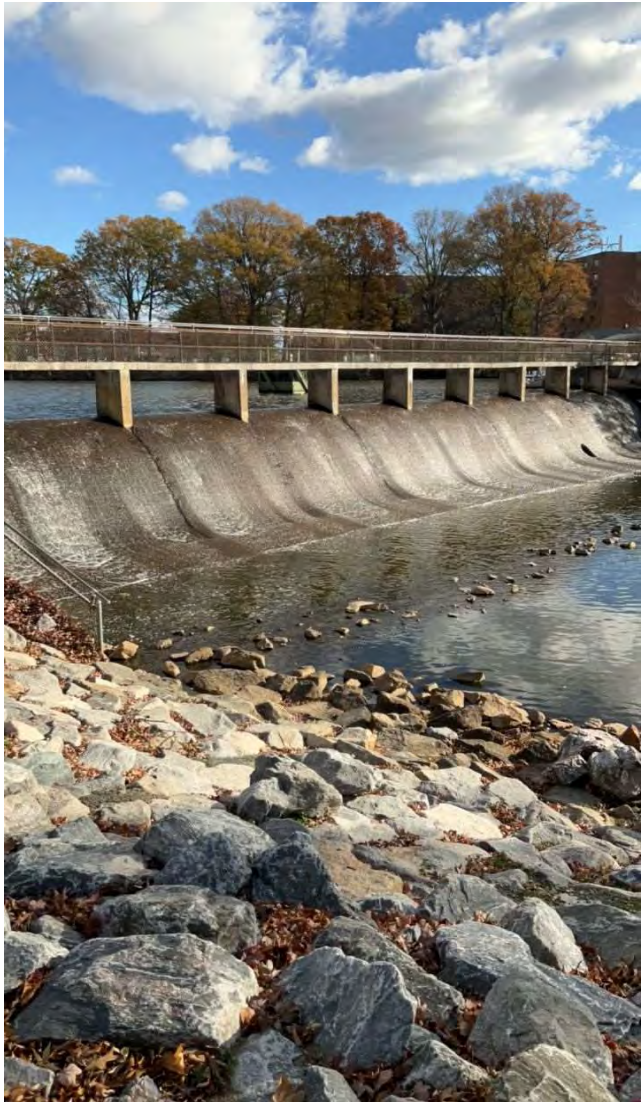
PHOTO 39: Overall downstream face of spillway.
