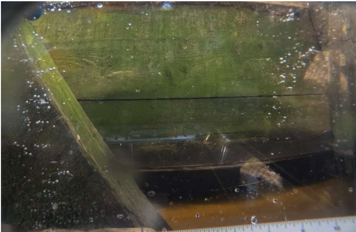
PHOTO 2: Timber cribbing around outlet works structure
