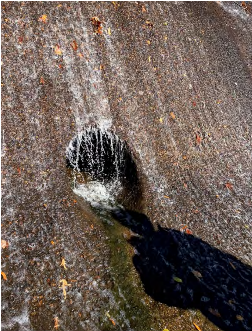
PHOTO 51: Outlet end of low level outlet works.
