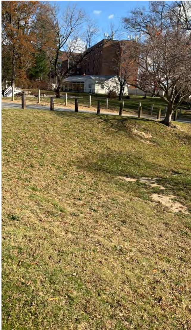
PHOTO 8: Downstream slope of left embankment.
