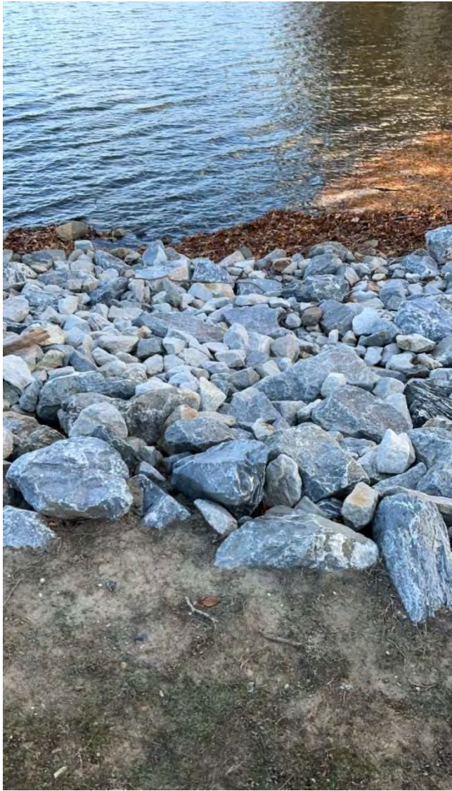
PHOTO 3: Typical riprap gradation along upstream slope east of boat ramp.
