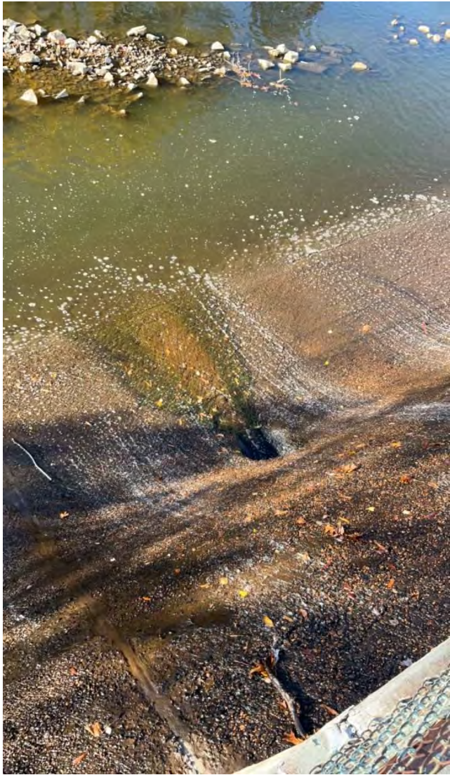
PHOTO 41: Overhead view of low level outlet works discharge through spillway.
