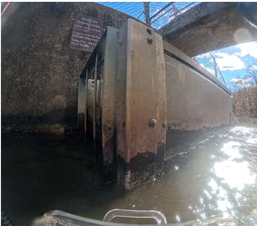
PHOTO 20: Fish ladder exterior framing
