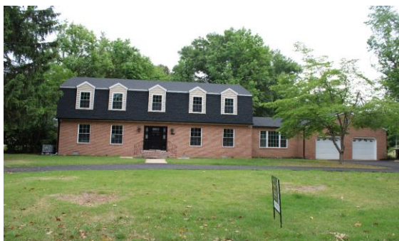
65 Laurel Drive - Major Renovations
