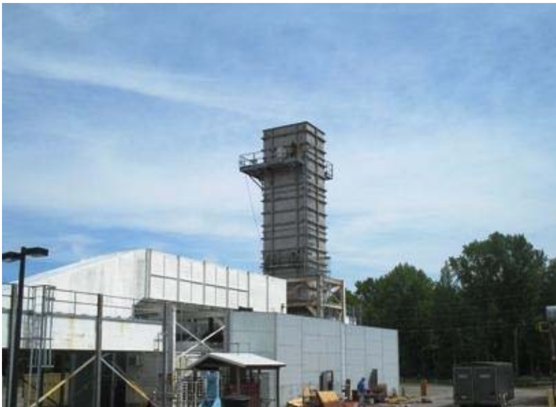
VanSant Generation Station Stack Repairs
