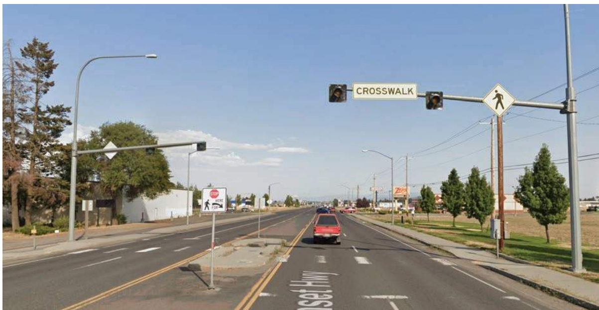
An example of a mid-block RRFB crossing with a pedestrian refuge island in Airway Heights, WA
