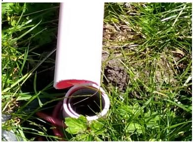
On June 1, 2019, Wayne Frey checked Country Glen Park Soccer Field and found that one of the goal posts has been broken near the base, which creates a safety hazard and non-functional goal post. Both goal posts are very weathered. The PVC pipe has faded from Red to White. The purpose of this request is to replace both goal posts and nets with a Matching Grant Program Application.
