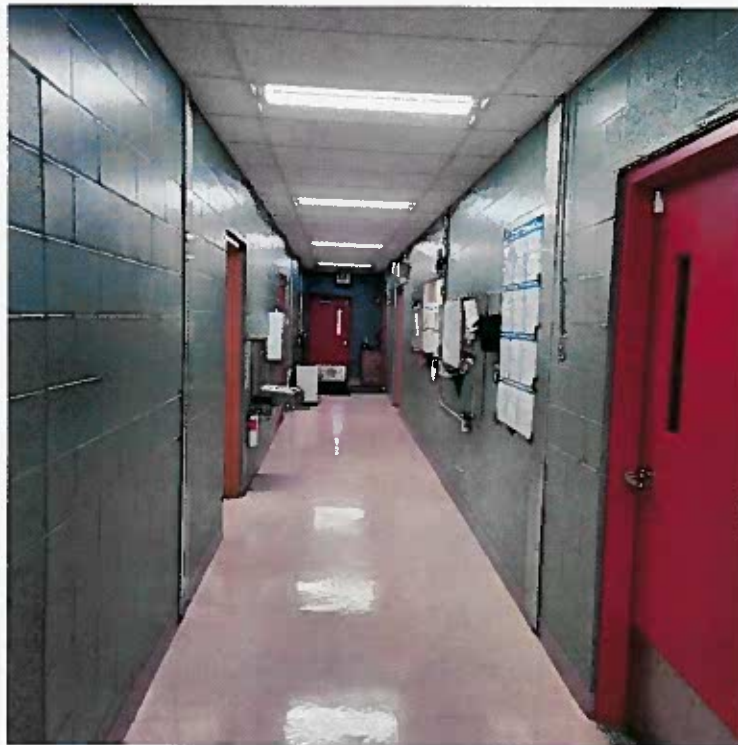
Primary Building Office Corridor
