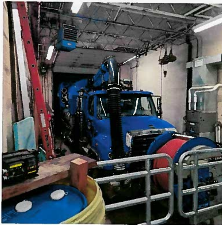
Primary Building Garage located off of Press Room
