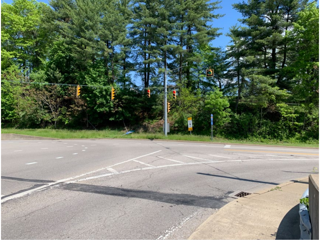
NB CR 70/1 (Washington Avenue) at I-70 WB On-Ramp
