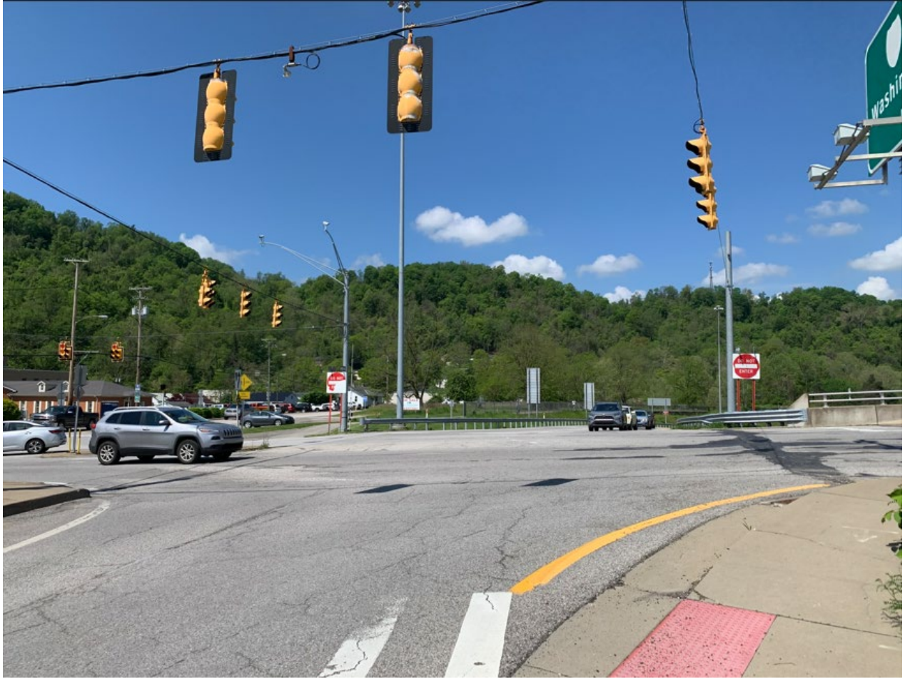
1-70 EB On-Ramp at CR 70/1 (Washington Avenue)
