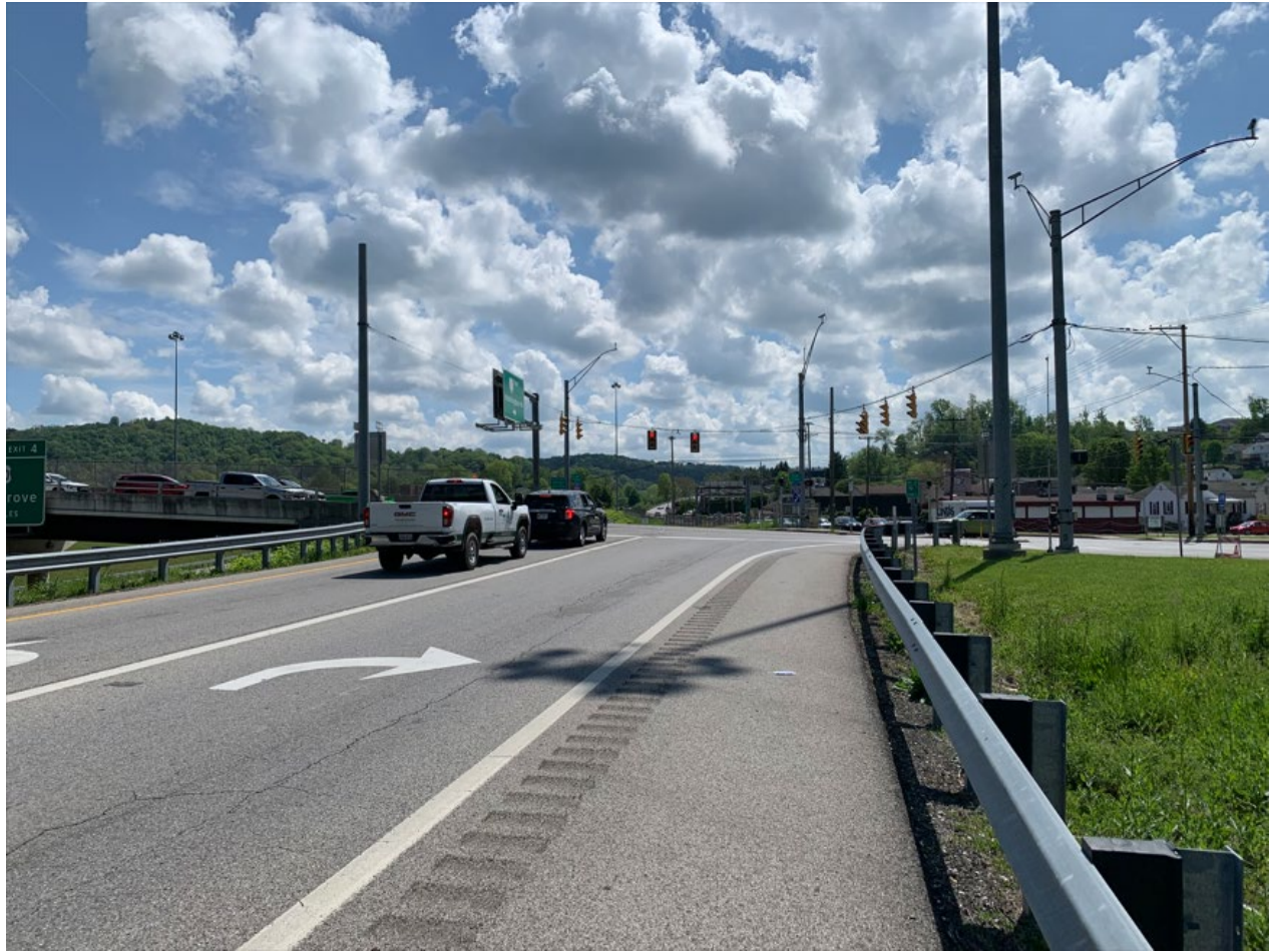
I-70 EB Off-Ramp at CR 70/1 (Washington Avenue)
