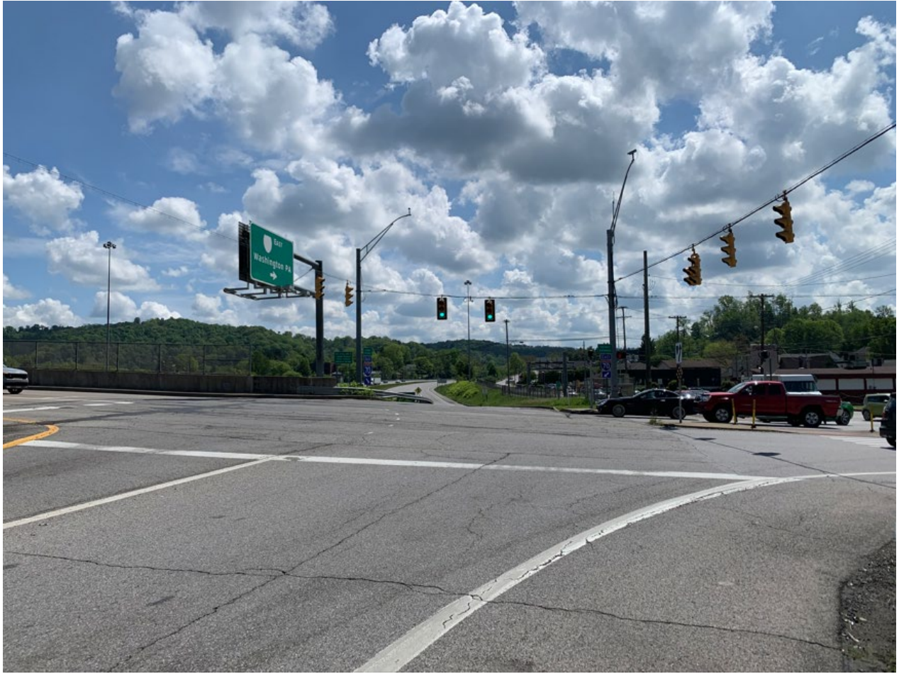
I-70 EB Off-Ramp at CR 70/1 (Washington Avenue)
