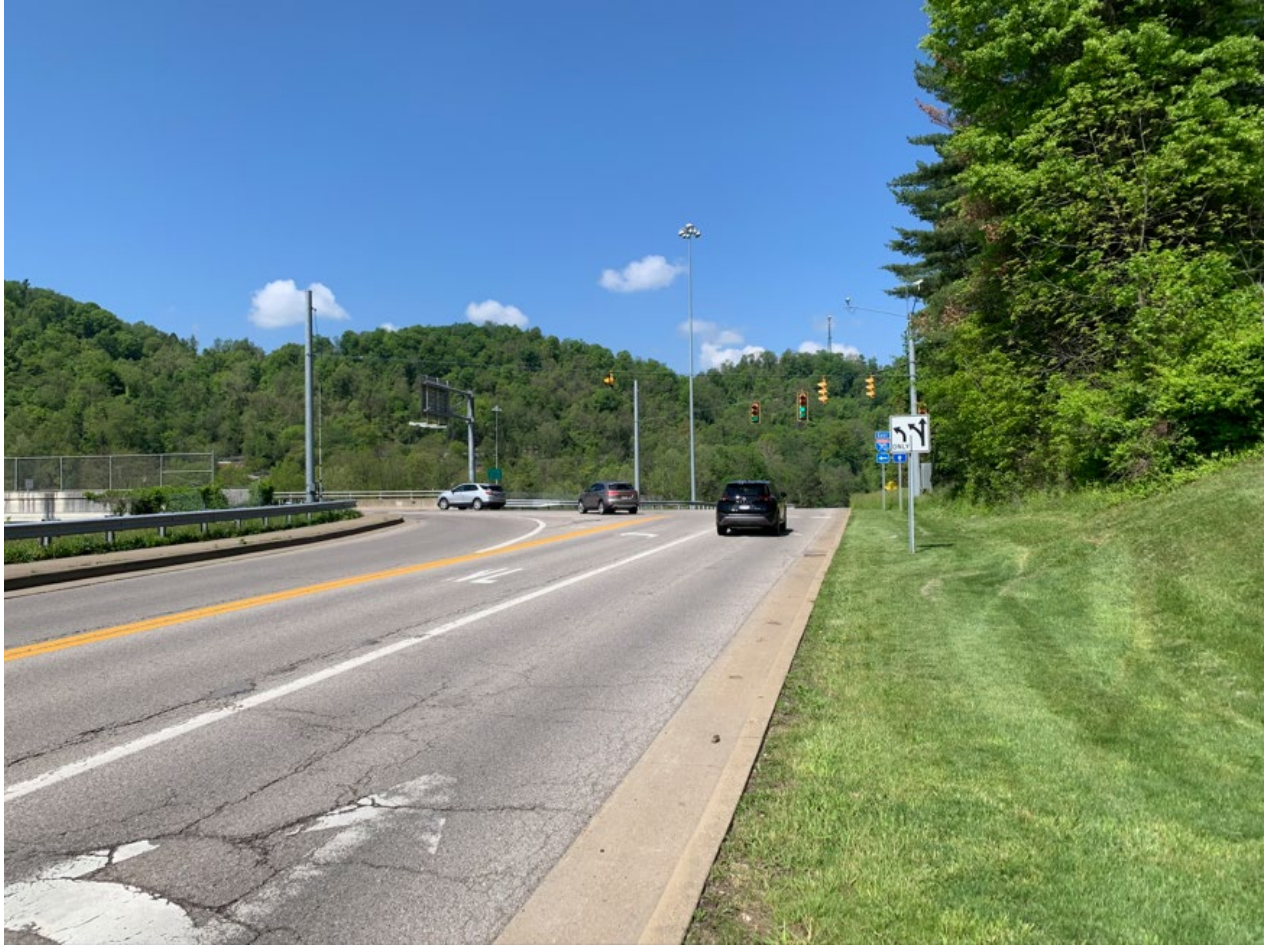
WB CR 70/1 (Washington Avenue) at I-70 WB On-Ramp
