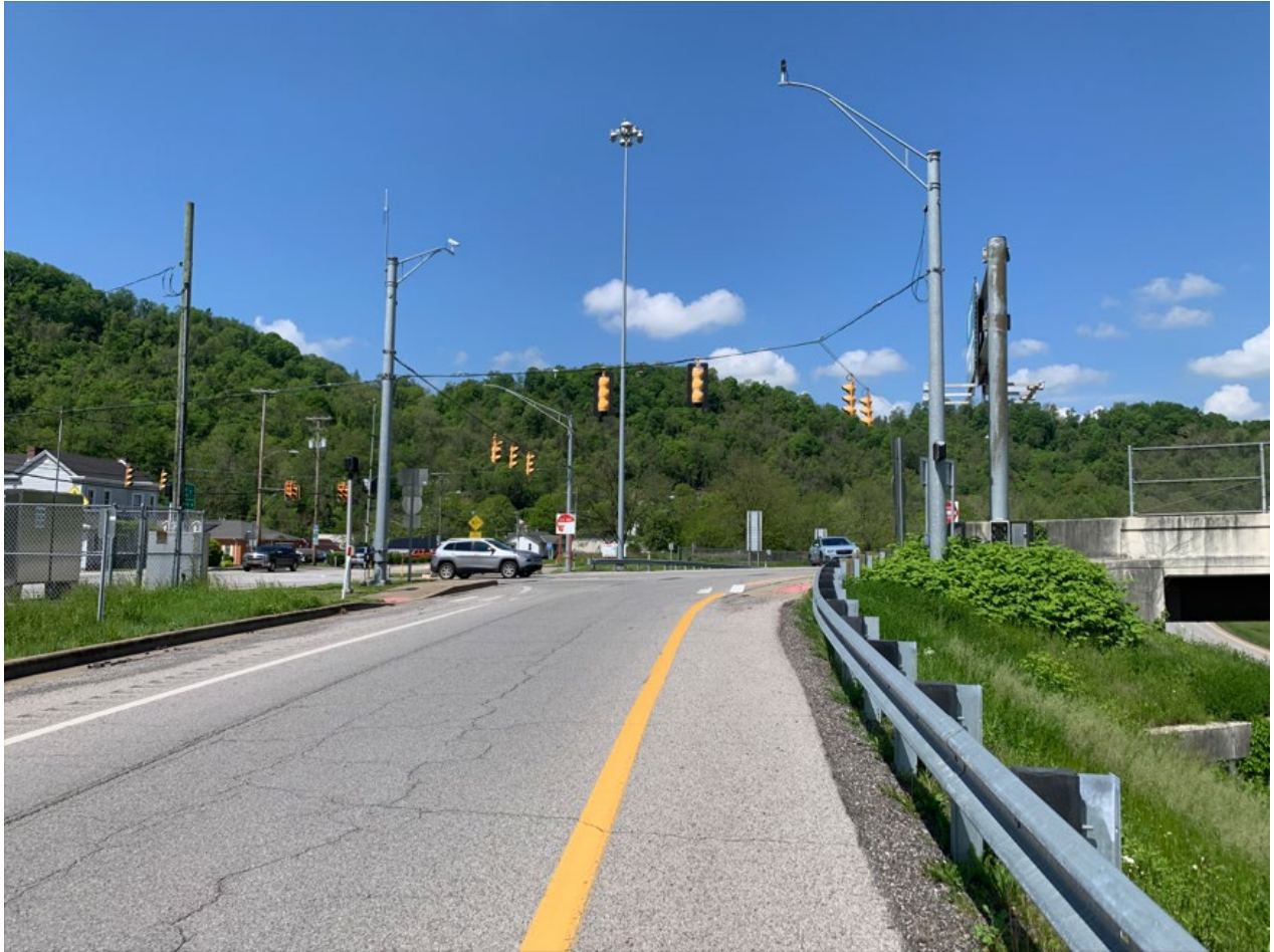
1-70 EB On-Ramp at CR 70/1 (Washington Avenue)
